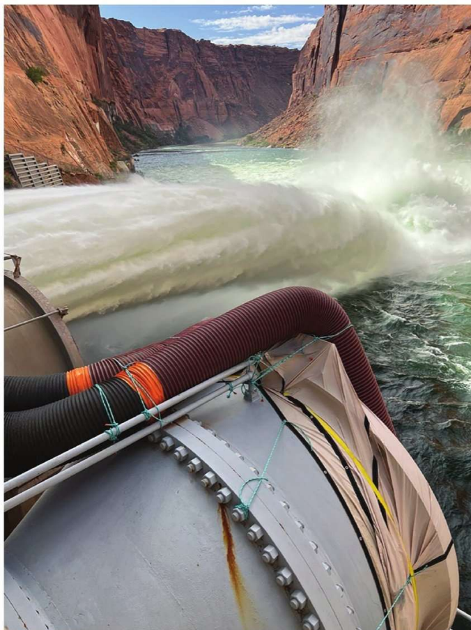
FIG. 4: One of the four bypass tubes currently under containment while robotic blast-cleaning takes place in the interior.
