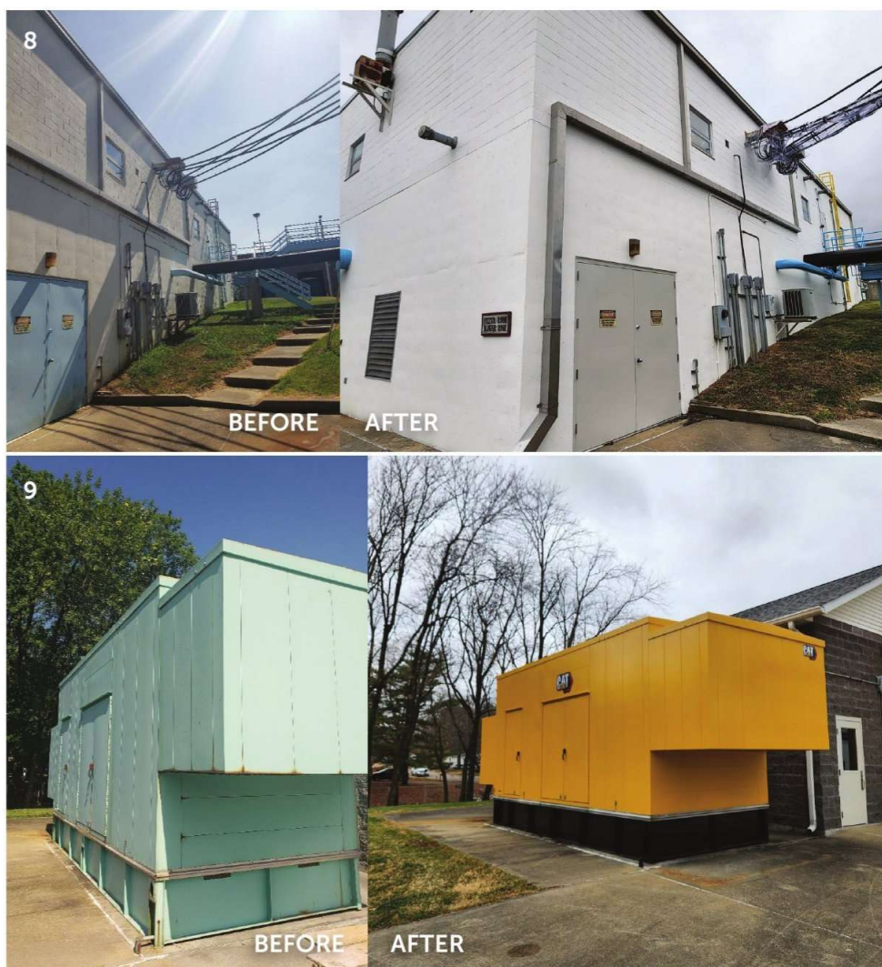
FIGS. 8 AND 9: Cementitious building surfaces and the facility generator were also coated to refurbish the facility's previously deteriorating conditions.
