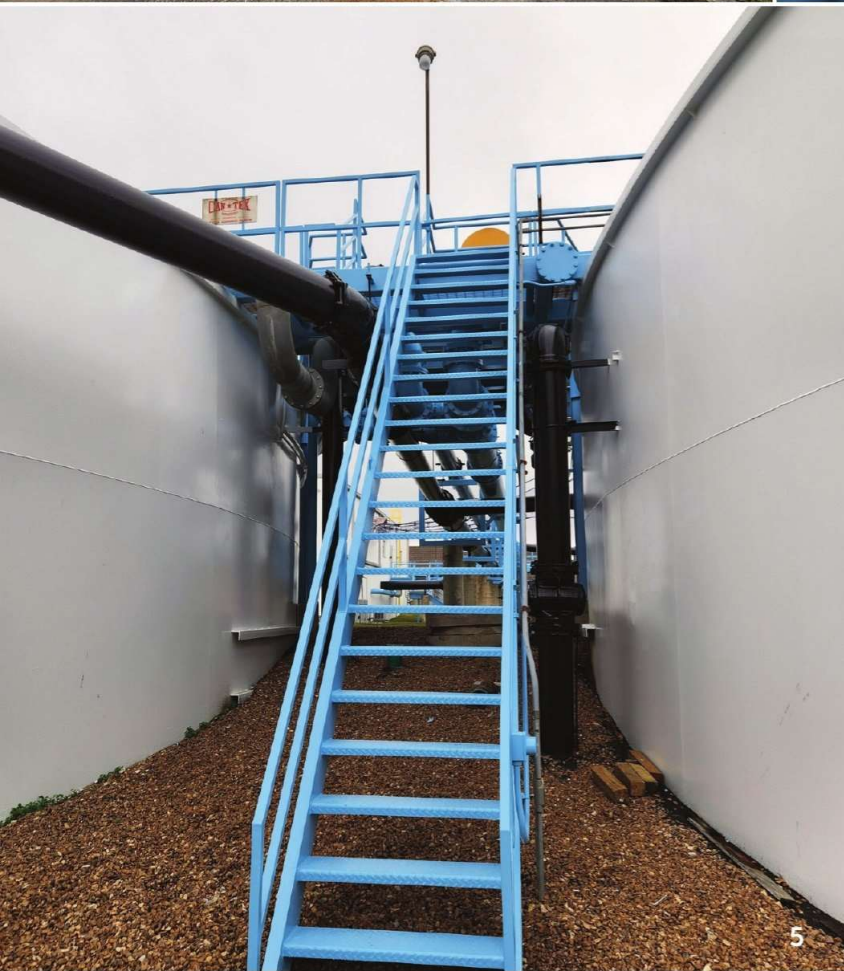
FIGS. 4-7: Various catwalks, stairways railing, piping and structural steel were recoated in the facility's exterior storage area and concrete basins.
