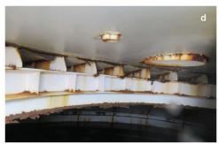
Prior to work taking place, readings were taken on the tank column referencing milage and cracking failure (a), while spot adhesion testing and milage readings were taken on the roof radial plate (b). Corrosion was widespread on the interior dry catwalk and access table (c) and the immersion compression ring (d). There were additional indications of a thinning coating system on the roof radial plates (e and f).
