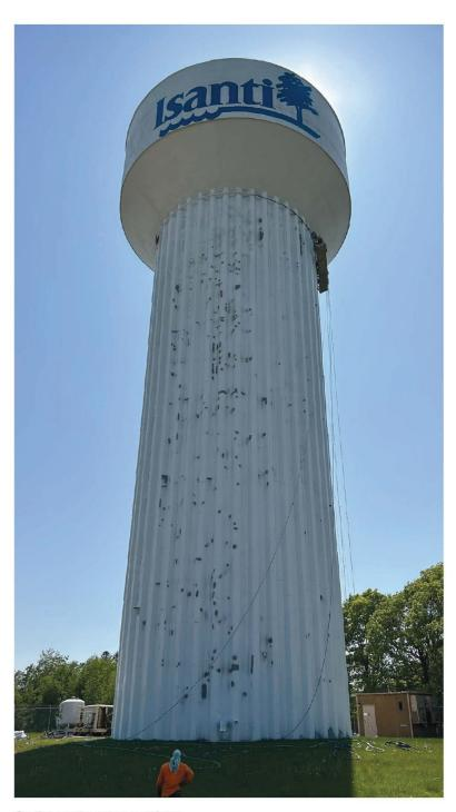
On the southeastern quadrant of the tank, numerous spots were abrasive blast-cleaned to a Commercial finish.
