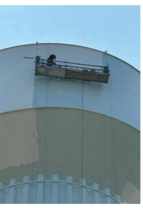
After primer application, an initial tie-coat of epoxy was applied to the tank's girder and shell plates.
