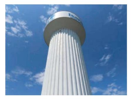
A polyamidoamine primer coating was applied across the previously blasted spots of the tank's fluted column.
