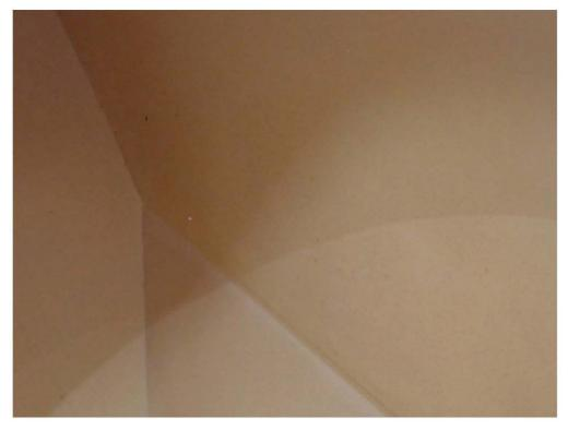
FIG. 4: A hybrid elastomeric polyurethane lining as seen five years after installation in a hopper car in salt service.
