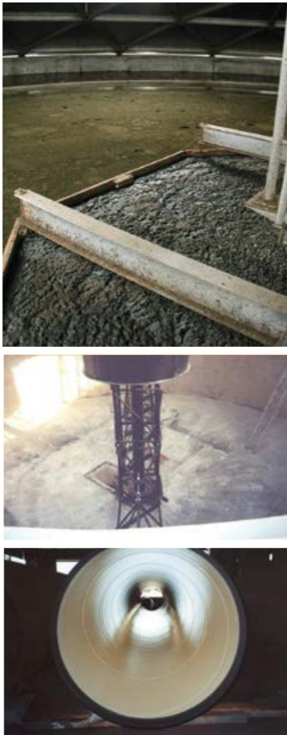
FIG. 6: Modified Epoxy Coating B2 was successfully applied in sewage plants (top and center); and for potable water service (bottom).
