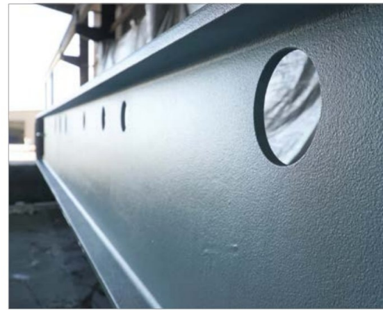
FIG. 7: Spraying fireproofing coatings inside a controlled shop environment enables applicators to achieve the best finish for Architecturally Exposed Structural Steel (AESS).
