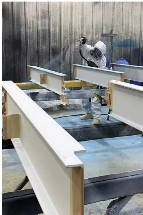
FIG. 3: Inside a shop, applicators can easily apply primer and then mask off holdback areas (3a) before spraying fireproofing coatings. On-site applicators will then fireproof those areas after the steel is integrated into the building's structure (3b).
