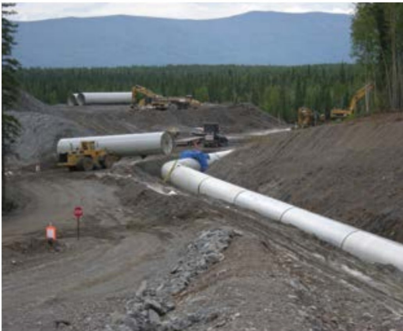
FIG. 3: Hydrocarbon-Modified Epoxy Coating A on penstock exterior.
