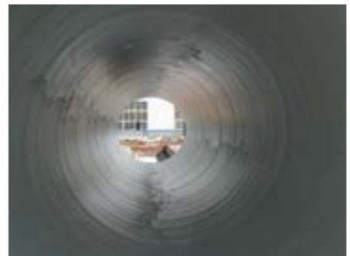
FIG. 4: Hydrocarbon-Modified Epoxy Coating A application in penstock interior.
