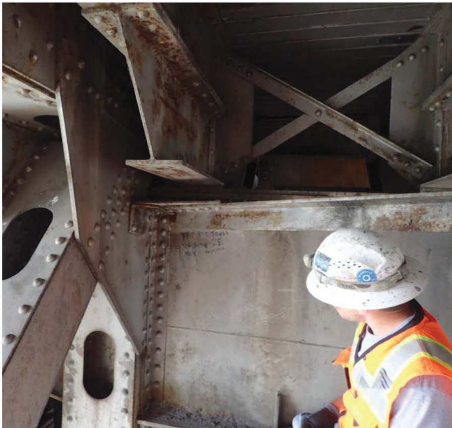
The bridge had not been painted since its original construction, and the steel and coatings were showing signs of deterioration.
