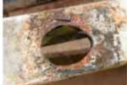
Fig. 3: Galvanic corrosion on rake arm mechanism
