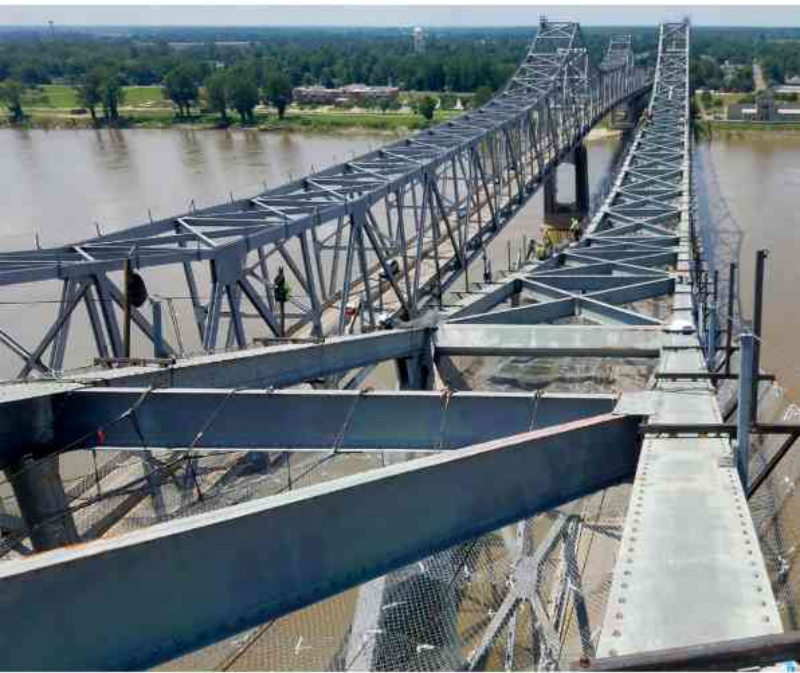
Safe bridge access was provided for painting, pin replacements and subsequent inspections.
