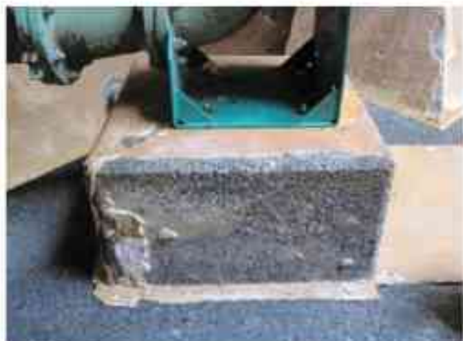
Fig. 5: Example of small exposed aggregate in immersed concrete exposed to FOG
