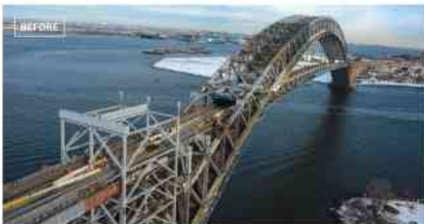
The roadway of the Bayonne Bridge had to be lifted in order to accommodate larger shipping vessels passing underneath. PHOTOS COURTESY OF AHERN PAINTING CONTRACTORS INC.
