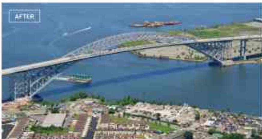
After a highly complex six-year rehabilitation project, the Bayonne Bridge's new roadway, protective coatings and related improvements were complete.
