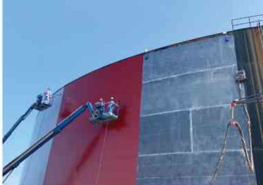
Fig. 3: UHP robotics can allow different work to take place concurrently, such as coating application taking place side-by-side with UHP waterjetting.
