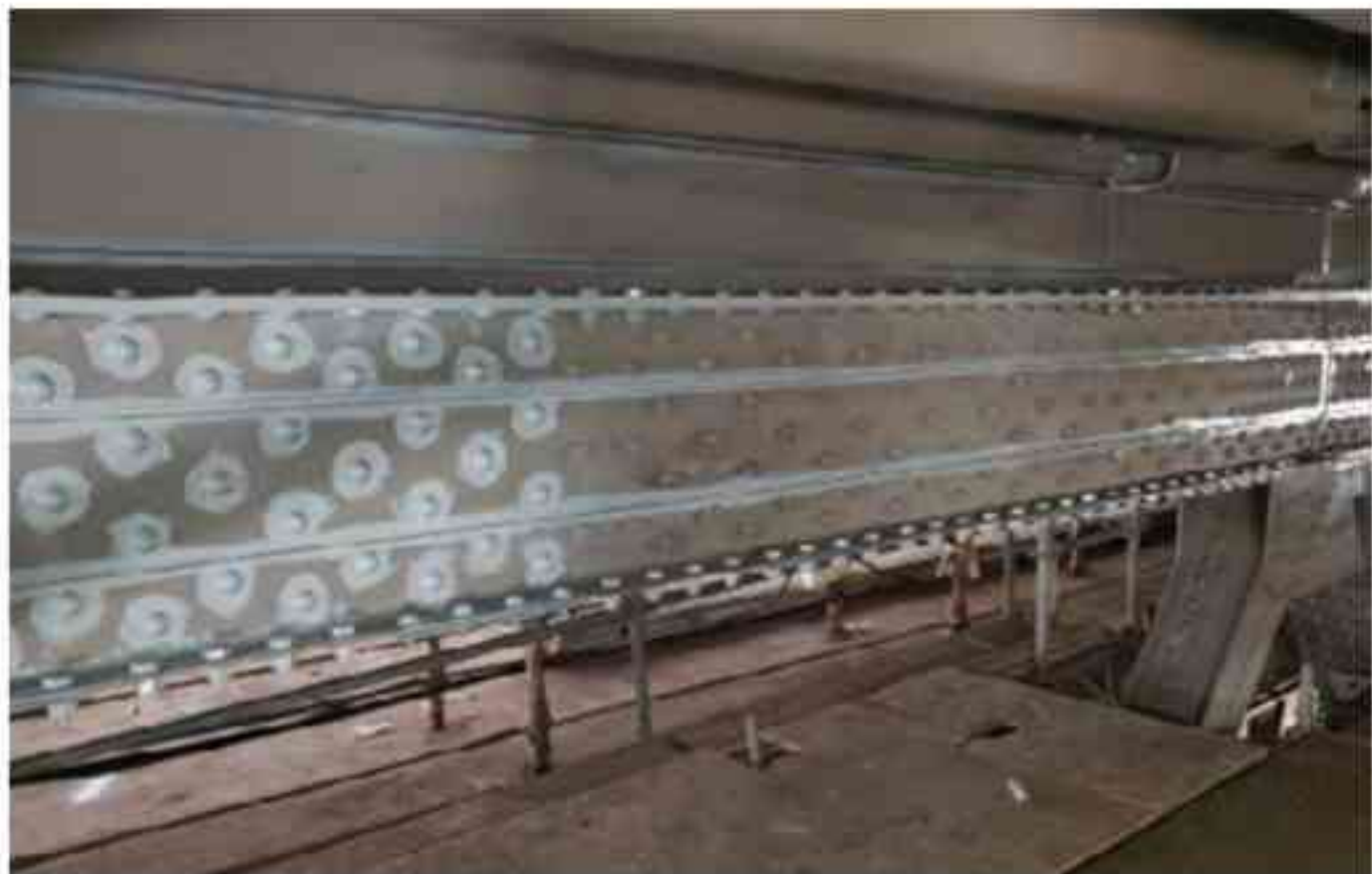
Fig. 4: Zinc primer and stripe coats applied.
