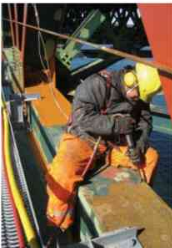
Fig. 1: Localized touch-up on the Macdonald Bridge. Photos courtesy of Halifax Harbour Bridges unless otherwise noted.
