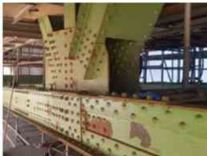
Fig. 2: Pre-blast condition.
