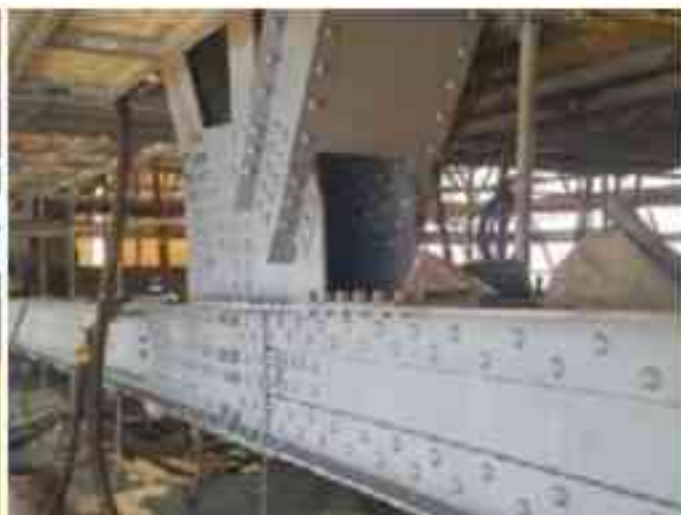
Fig. 3: The existing steel was pressure-washed and blast-cleaned to SSPC-SP 10/NACE No. 2.
