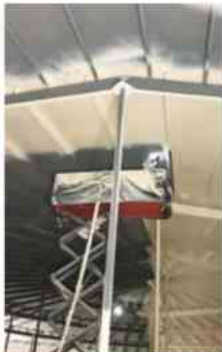
Fig. 3: Elastomeric polyurethanes serve well on lap seams on tank ceilings due to their excellent elongation properties, often allowing applicators to skip caulking seams.
