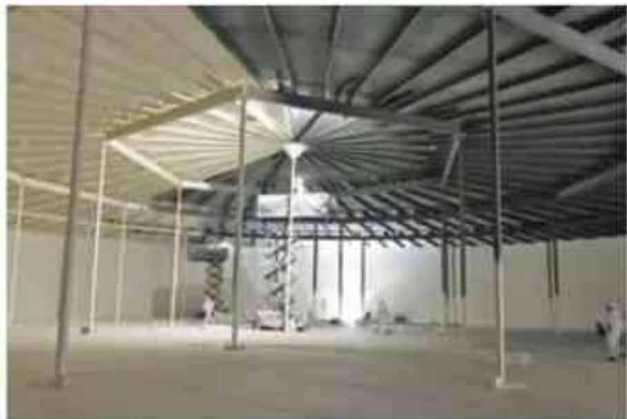
Fig. 2: Applicators can achieve film builds of up to 350 mils' (¼ inch) DFT when spraying elastomeric polyurethane linings.
