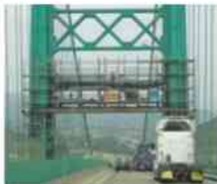
Beams traversing roadway for upper tower scaffolding support. Photo courtesy of Caltrans.
