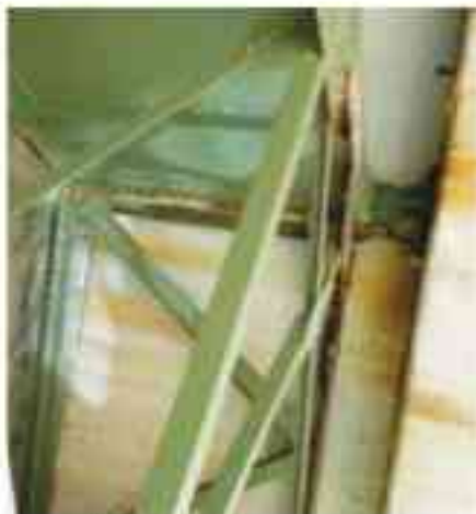
Coating System J, the elastomeric acrylic, showed blistering, peeling and corrosion on approximately 20% of the total surface area. Photos courtesy of the author.
