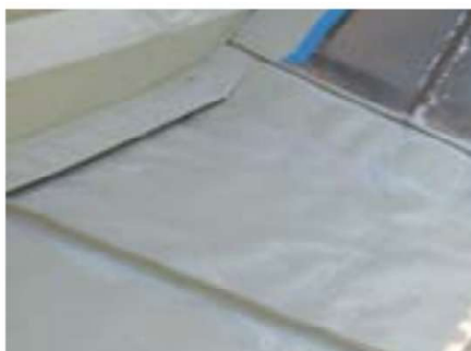
Fig. 4: Thin-gauge metal raised-seam roofing panels that buckled as a result of abrasive blast-cleaning.
