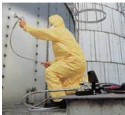
Fig. 2: If spraying in hard-to-reach areas or tight spaces, selecting a machine that is on a cart and easy to move might be of importance.
