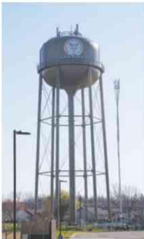
The 5,000-gallon tank was pressure washed and topcoated, saving the owner the cost of a full blast and recoat. Photo courtesy of City of Oak Grove.
