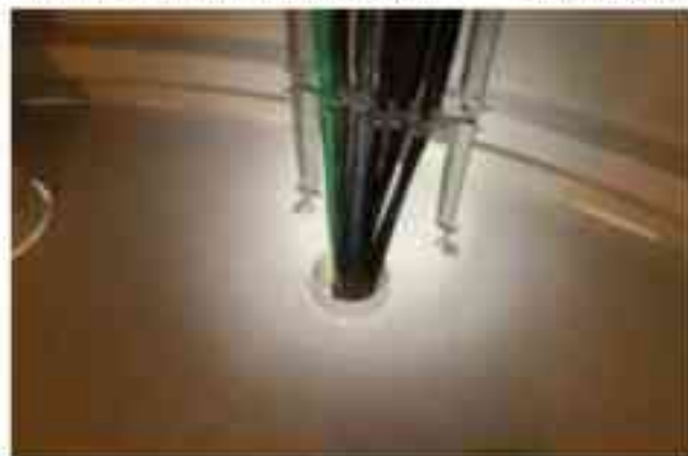
Fig. 6. Painted welded water tank platform penetration.
