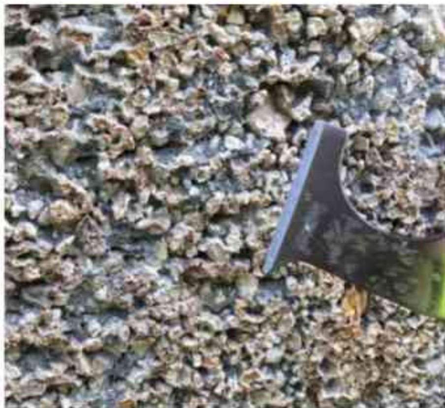
Fig. 1: Existing cast-in-place concrete surface following surface preparation. Figures courtesy of the author.
