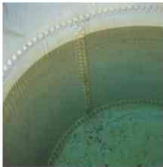
Fig. 3: A riveted water tank lined by the author more than 25 years ago remains in pristine condition. This tank is well over 100 years old and had exhibited severe corrosion. Blasted to SSPC-SP 5/NACE No. 1, a thick-build coating system was applied. Twenty-five years later, there's not a single holiday or any evidence of corrosion.
