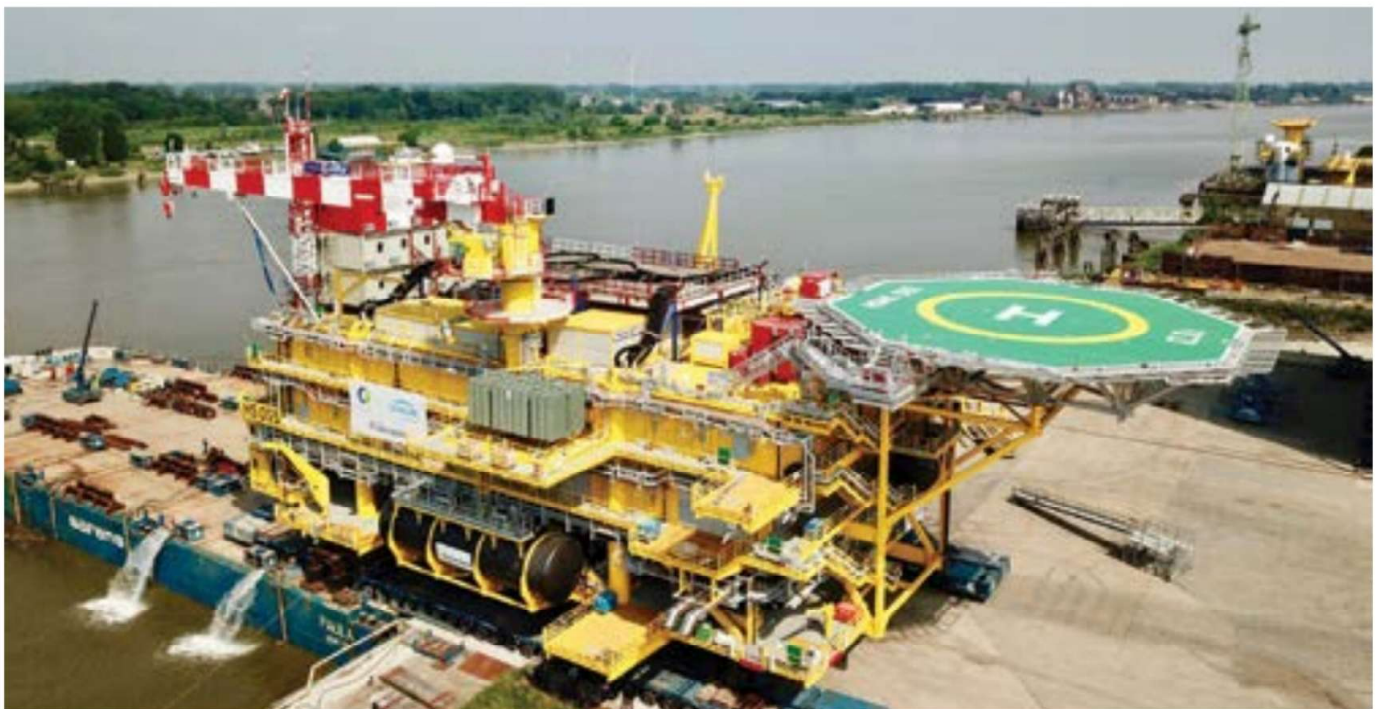
Fig. 4: The 55-meter-long, 30-meter-high substation totaled over 4,500 tons in weight.
