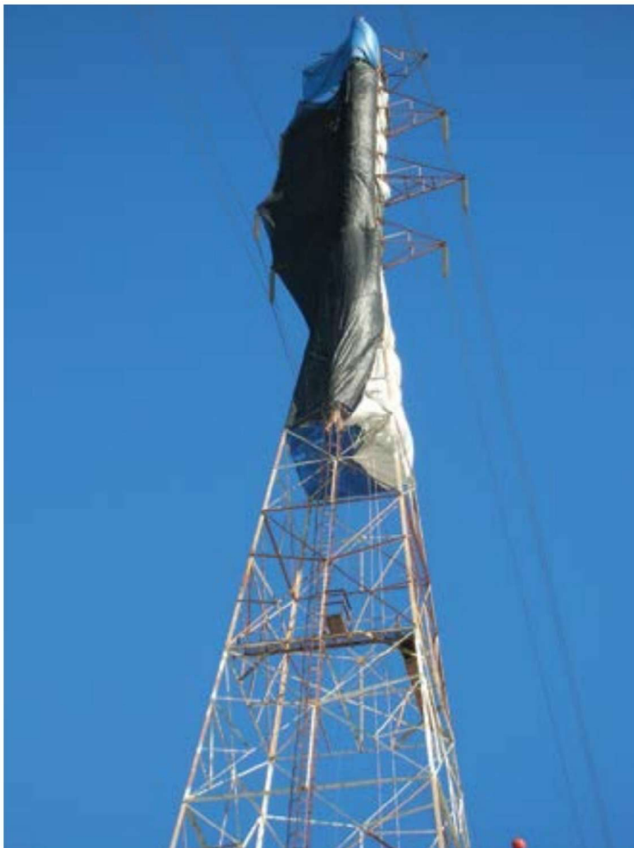
Fig. 2: The enclosure structure was moved down the tower as the work progressed and was lowered to the base of the tower at the end of each day.
