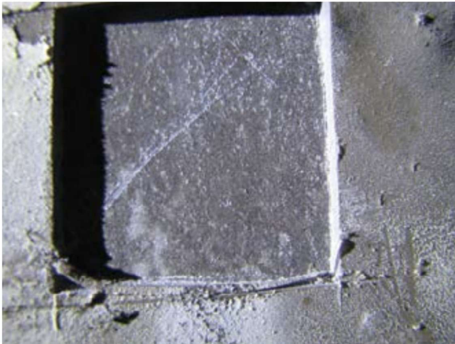
Fig. 5: In areas well above the waterline, the primer and polyurea coating were in good condition
