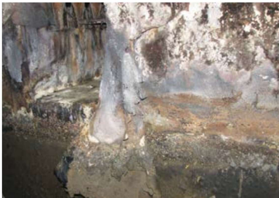
Fig. 2: Delaminating coating around a penetration in a CEPT area.
