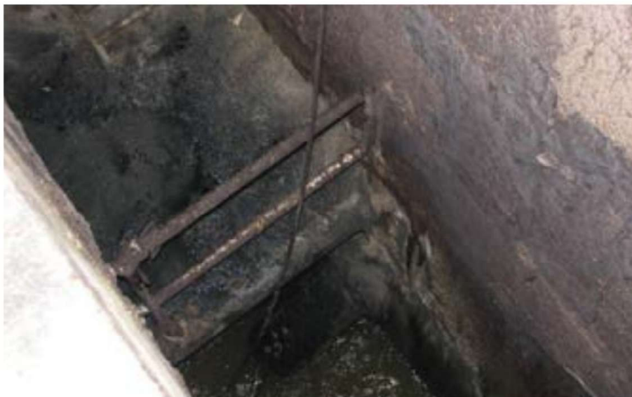
Fig. 1: Concrete was degraded in an unventilated manhole. Photos courtesy of KTA-Tator, Inc.
