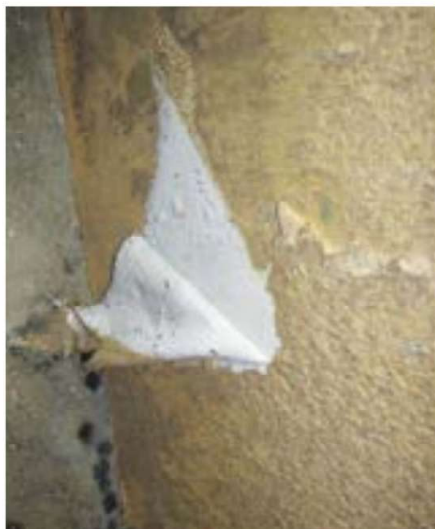
Fig. 3: Poor adhesion between two coats of polyurea.
