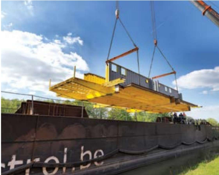
Fig. 3: Individual components were fabricated and coated at different facilities, then transported to a separate site for construction.
