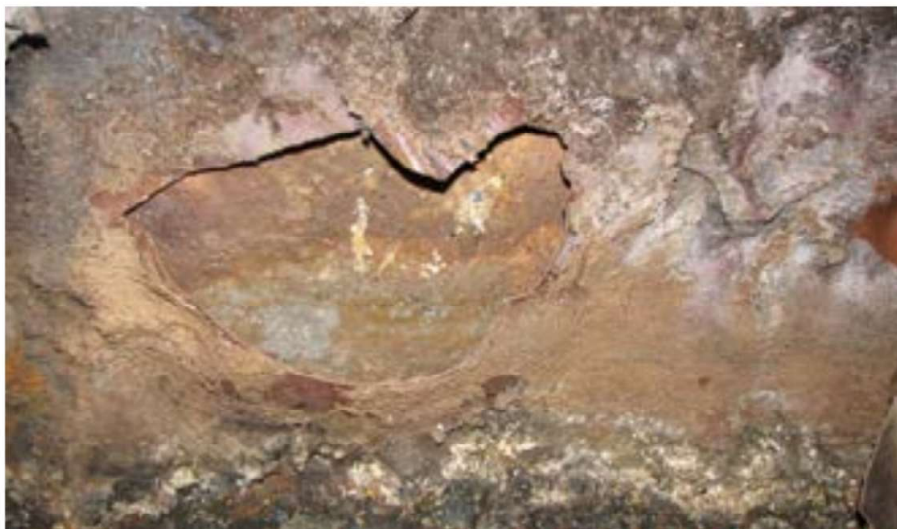
Fig. 4: Delamination and discoloration above the waterline.
