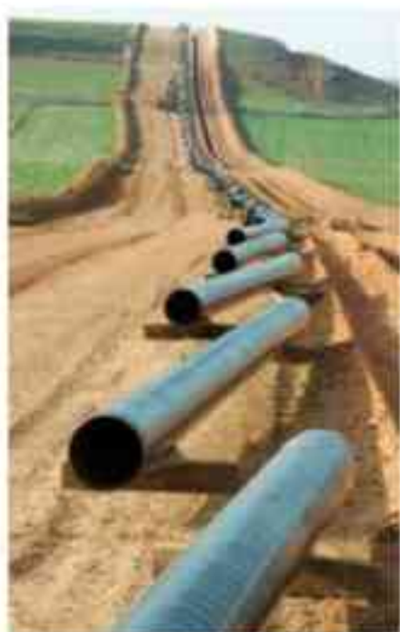
Fig. 5: An abrasion-resistant coating will help protect pipes from scratches and scrapes as they're dragged across soil and gravel during installation and operation.
