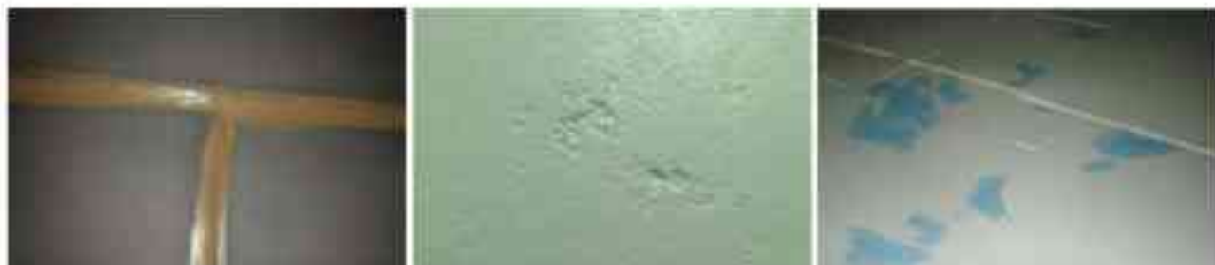
Fig. 11 (L to R) Stripe coat with solvent-borne epoxy holding primer, full application of the holding primer and pits filled flush with epoxy caulk. Right-hand photo courtesy of Rick Jondreau, M.R. Consulting Inc.
