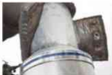
Fig. 4. Removable, reusable insulation blankets with flexible jacketing on both sides allow removal, replacement and inspection of the entire area under the blanket.
