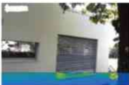
Fig. 9: An area of blistering in an applied coating is detected by the IR-TI image on the right.
