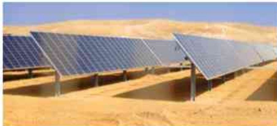
Fig. 1 Many solar projects are located in arid, desert regions where the soil may present corrosive conditions for underground steel structures. (Photo: Getty Images / Edward Leyens)
