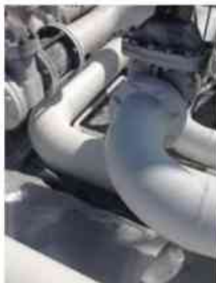
Fig. 6: A spray-applied insulative coating is helping to minimize burn hazards to personnel, as well as maintain the external temperature of this crude-oil pipeline, which operates at 180–260 F (82–93 C) with spikes to 350 F.
