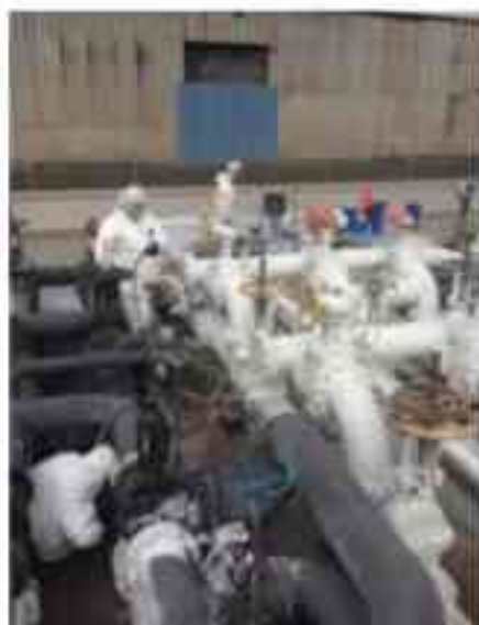
Fig. 6: A spray-applied insulative coating is helping to minimize burn hazards to personnel, as well as maintain the external temperature of this crude-oil pipeline, which operates at 180–260 F (82–93 C) with spikes to 350 F.
