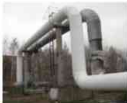
Fig. 2: Using a thermal insulative coating (left) on processing ductwork prevents the hidden and costly threat of CUI that comes from using traditional insulation and cladding systems (right).
