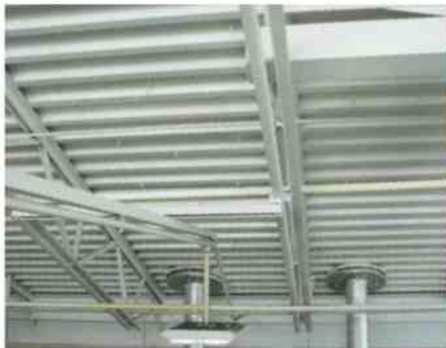
Fig. 1: View of the interior roof from ground level. Photos courtesy of KTA-Tator, Inc.
