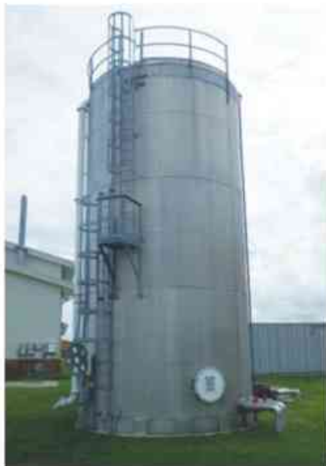
Fig. 1: Water-storage standpipe with aluminum jacketing. Photos courtesy of the U.S. Navy.
