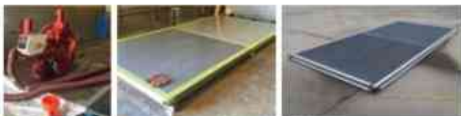
Fig. 6: (From left) Surface preparation, primer application and nonskid application.
