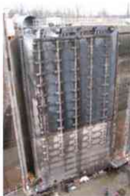
Fig. 1: Miter gates from the Welland Canal with a vinyl coating system. Photos courtesy of KTA-Tator, Inc. unless otherwise noted.
