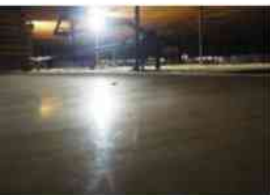
Fig. 1: Light reflects off a 25-year-old epoxy lining that protected a 150-foot-diameter tank floor from internal corrosion. Photo courtesy of Enbridge.
