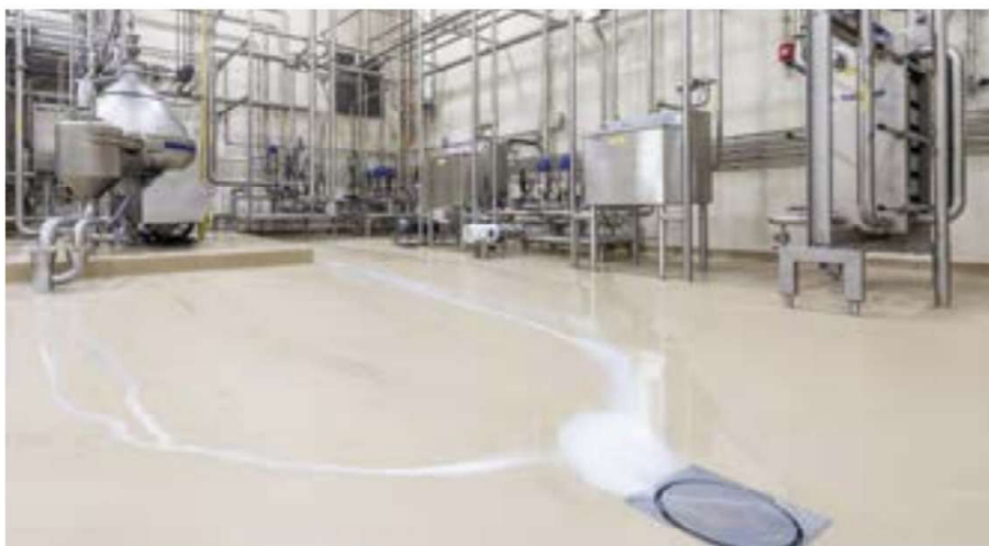
Fig. 3: The industrial floor coating system had to be resistant to cleaning agents as well as intermittent contact with milk products.
