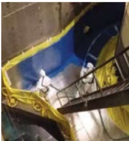
Fig. 7: Workers apply polyurea in the reactor cavity.
