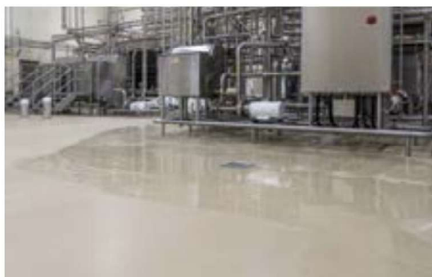
Fig. 2: Water from the sterilization process flows over the flooring system and is collected for treatment and agricultural reuse.
