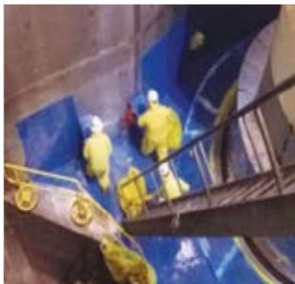
Fig. 8: Workers remove contaminated polyurea in sheets from the reactor cavity walls and floor.
