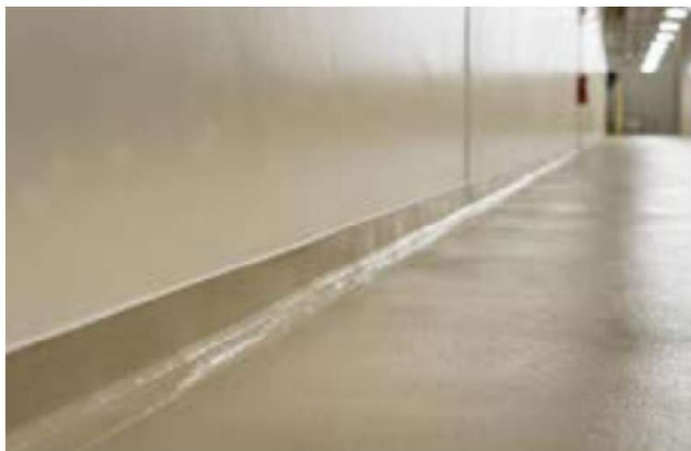
Fig. 5: Over 14,000 linear feet of cove base was created using a polyurethane mortar and a polyaspartic-based topcoat.
