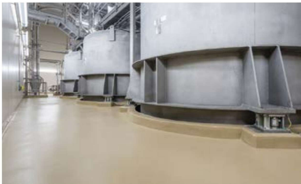
Fig. 1: The area around the large storage tanks required a protective coating on the floor as well as on the cove base areas and curbs. Photos courtesy of T.W. Hicks Inc.
