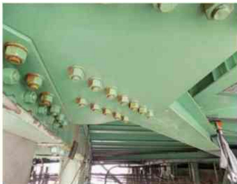
Fig. 2 Bolts rusted after improper preparation.
