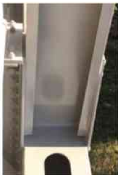
Fig. 5: All coats, caulking and stripe coat of finish applied.
