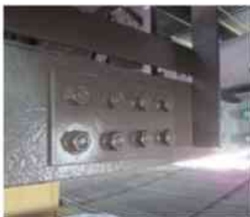
Fig. 4: A completed repair done correctly.
