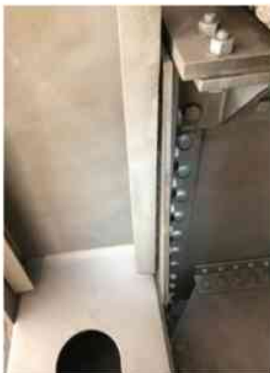
Fig. 3: Typical removal of pack rust by blast cleaning.
