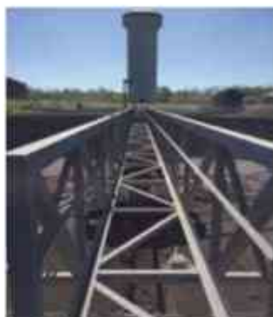
Fig 1: Clarifier barge structure. Photos courtesy of the author.
