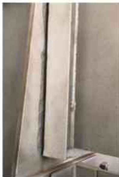
Fig. 4: Typical removal of pack rust by blast-cleaning.
