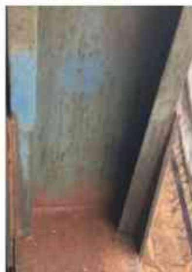
Fig. 2: Prior to blast-cleaning.
