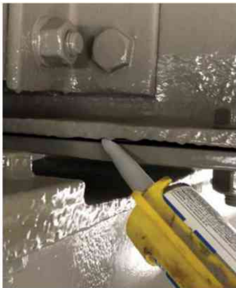
Fig. 6: Finish coat applied prior to caulking.
