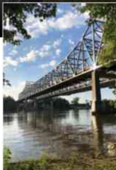
Fig. 1: Shade-Lohmann Bridge. Figures courtesy of the authors.
