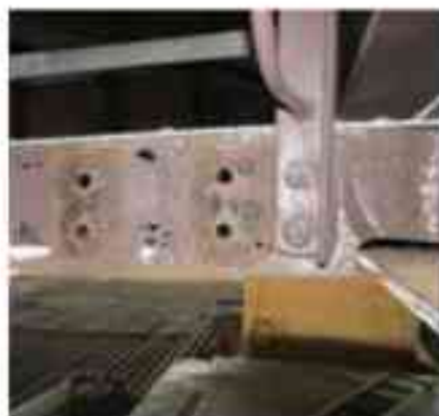
Fig. 5: Faying surface locations.
