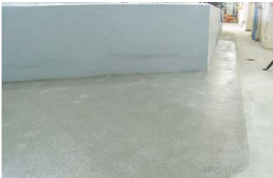
Fig. 4: No reflective cracking and no moisture-related problems have been observed since this floor coating was installed in a building at a wastewater treatment plant after two years in service. Photo courtesy of the author.
