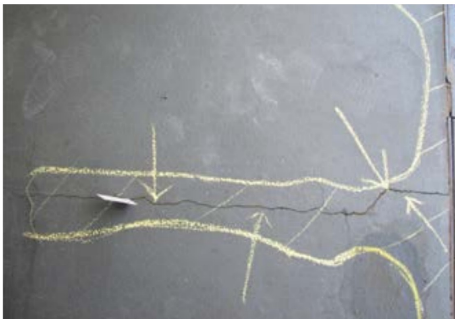
Fig. 3: Reflective cracking which appeared approximately one month after a floor coating system was installed in a pharmaceutical plant. Photo courtesy of the author.
