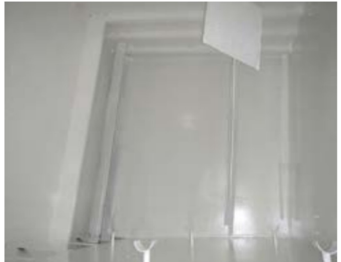
Figs. 4 and 5: An epoxy coating was applied at a 20-to-30-mils DFT over all the fish hold surfaces, including sharp edges, corners and grates.
