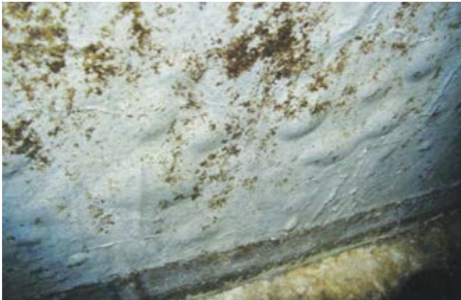
Fig. 5: Blisters formed in the coating on concrete walls in a wastewater treatment plant only two months after installation. Photo courtesy of the author.
