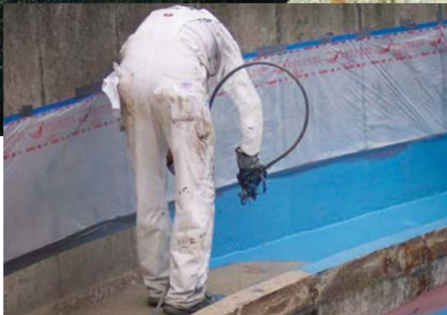
Fig. 1: Application of ceramic epoxy coating. Photos courtesy of Induron Protective Coatings.
