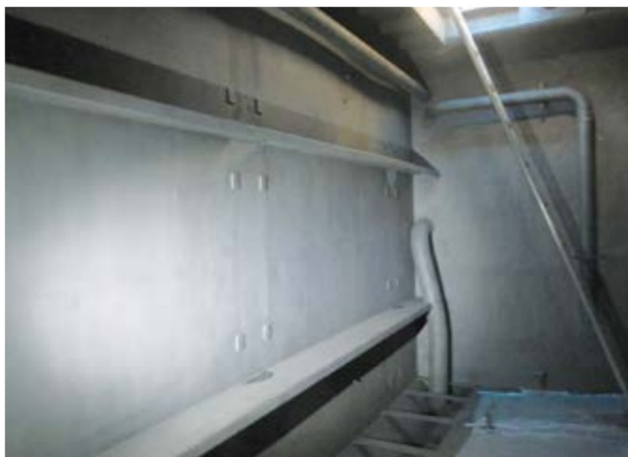
Fig. 3: Abrasive blast-cleaning the fish holds to an SSPC SP-10 standard removed all coatings and contaminants from the steel substrates.
