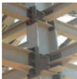
Fig. 9: Epoxy-polysulfide PFP applied to structural steel.
