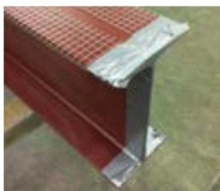
Fig. 8: Clip-on mesh on flange tips.
