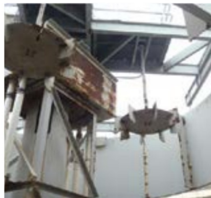
Fig. 2: This photo shows below-waterline corrosion at areas of coating failure.
