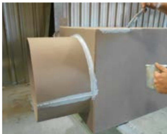
Fig. 4: Stripe coating the edges and corners is highly recommended to assure that good film quality and necessary film thickness are achieved.
