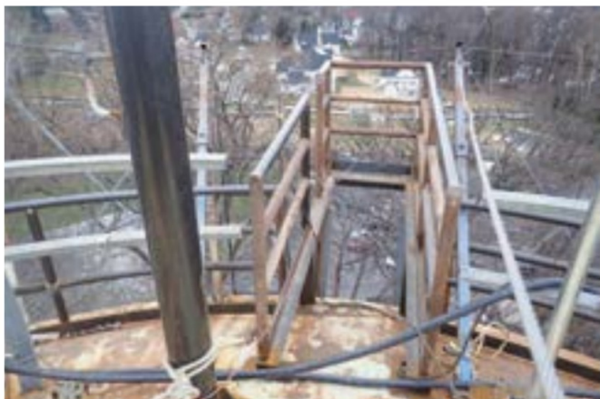
Fig. 2: The proposed improvements included new manways for improved internal access and confined-space access, a new roof ladder access system with resting platforms, new circular roof guardrails, a frost-resistant roof vent and other miscellaneous items.
