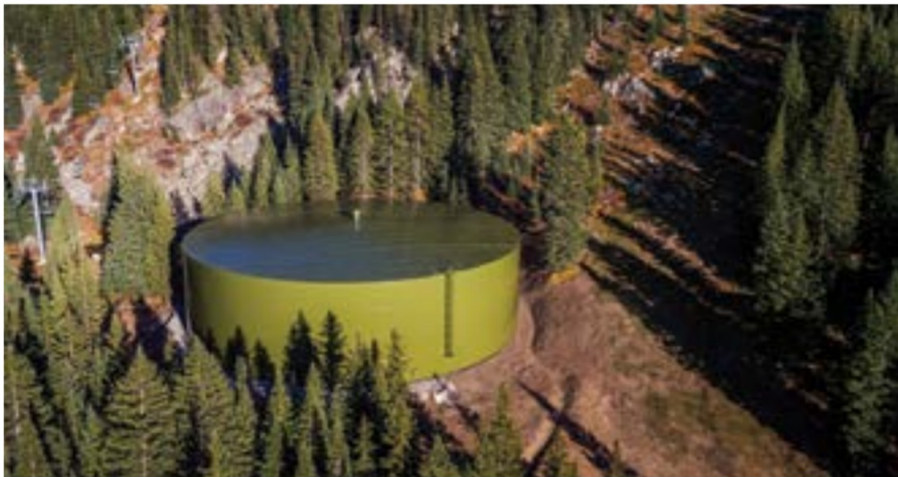
Fig. 3: Using a primer with a long recoat window and fast-cure intermediate and finish coatings helped the contractors overcome some of the project challenges.
