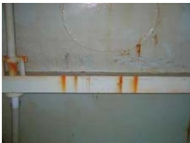
Fig. 1: Initial coating deterioration at weld beads and edges. Figures courtesy of the authors.
