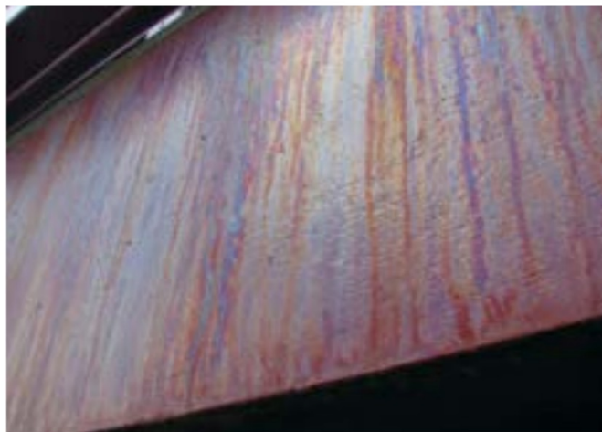
Fig. 4: Severe staining on north fascia.
