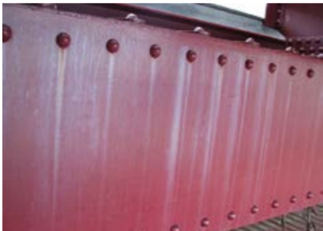
Fig. 3: Staining on north box chord.
