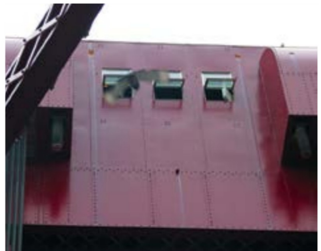
Fig. 2: Streaks of staining on one of the bridge lift towers.
