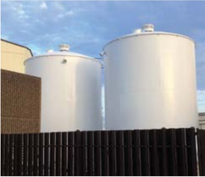
Fig. 4: Because the tanks were located about 50 feet from the flight line and in between two large hangers at a very active Air Force training base, wet abrasive blasting was chosen to avoid dusting out the facility, the other trades and possibly even the neighbors in the process.
