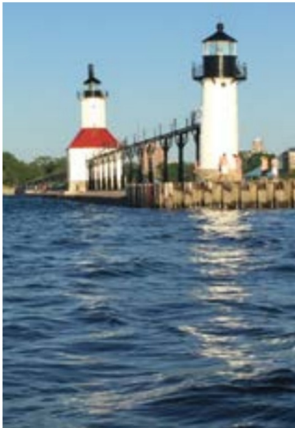
The 100-plus-year-old St. Joseph North Pier and Lighthouse was topcoated with a novel two-coat polysiloxane developed by the U.S. Naval Research Lab. Photo courtesy of NCP Coatings Inc.
