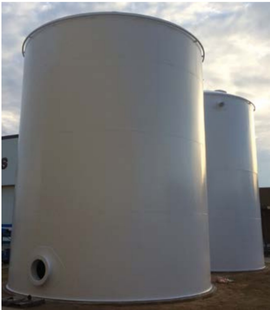
Fig. 1: This project involved recoating the interiors and exteriors of two ground storage tanks used by the U.S. Air Force to store water for firefighting. Photos courtesy of ICCI, Inc.
