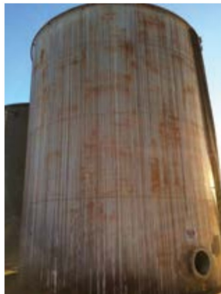
Fig. 2: Although the interior tank coating was considered preventative maintenance, the exterior was prematurely failing due to an adhesion issue.
