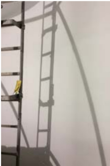
Fig. 3: A three-coat AWWA-compliant coating system consisting of a zinc-rich primer and two coats of epoxy, plus a stripe coat was used to line the tank interiors.
