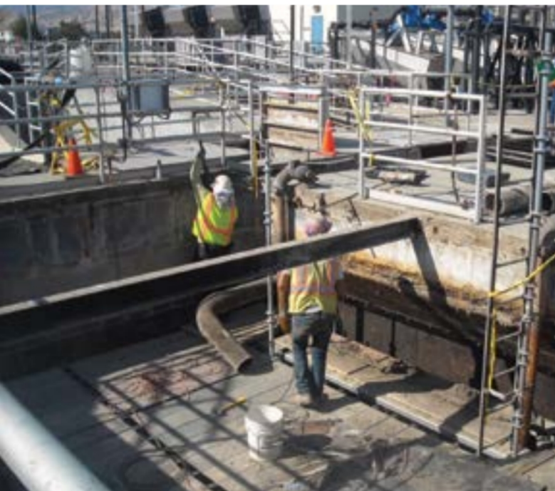
Fig. 2: The contractor begins work removing the lining system to uncover extensive H_2S damage.
