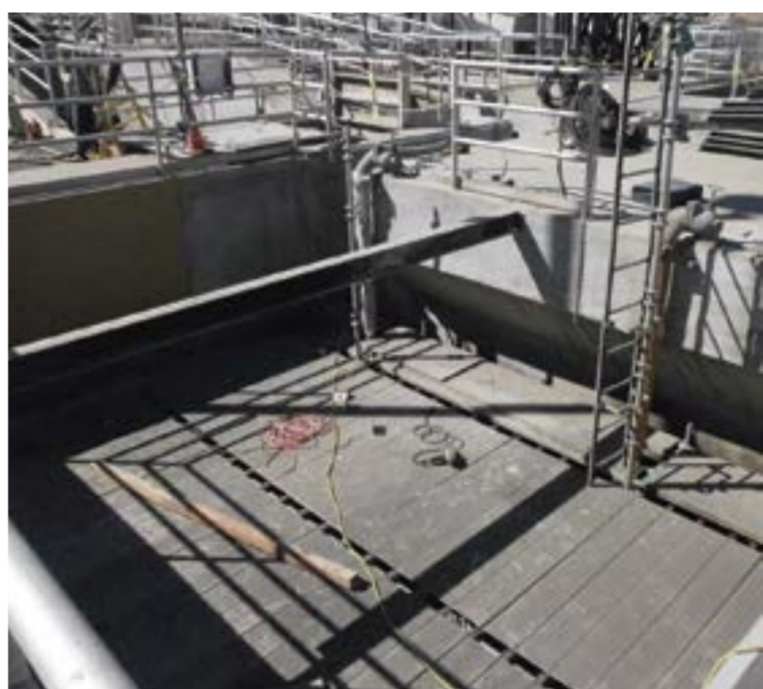
Fig. 3: The finished project used calcium aluminate cement.
