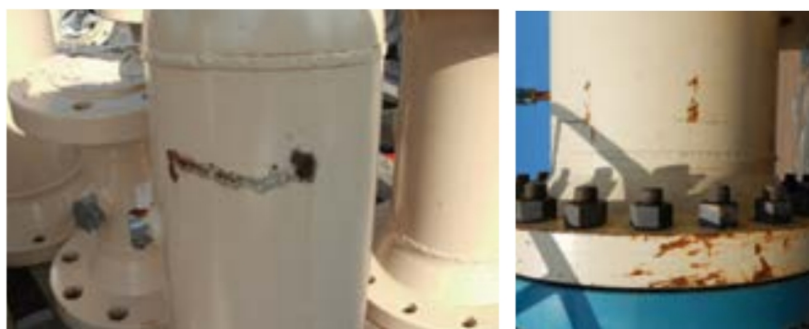
Fig. 3: Mechanical damage was evident on piping, flanges and structural steel after erection
