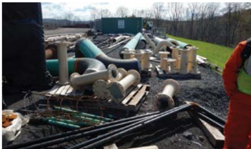
Fig. 1: Piping and structural steel were stored in a lay-down area prior to erection. Photos courtesy of KTA-Tator, Inc.
