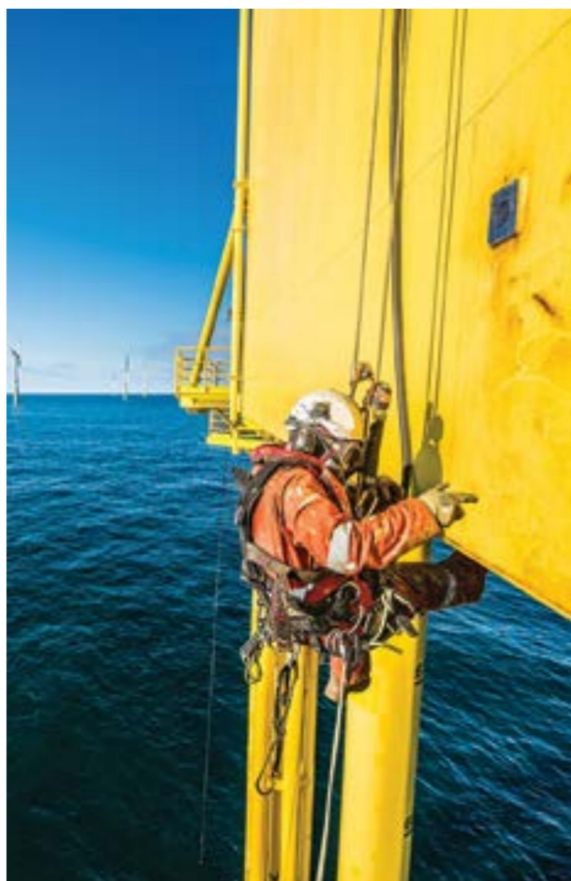
Fig. 2: Suspended from a main and a backup line, a rope access technician inspects the surface of a substation, a structure built in the Netherlands and installed on an offshore wind farm in German waters. Photo courtesy of Height Specialists.
