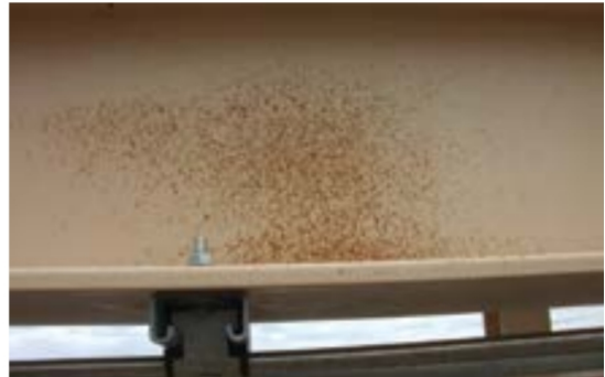
Fig. 4 (Clockwise from left): Pinpoint corrosion was observed on the piping, structural steel and flanges. Note that these surfaces were not abrasive blast-cleaned.
