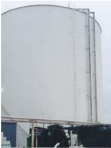
Fig. 3: A side view of the Behemoth. The tank was constructed of steel nearly an inch thick.
