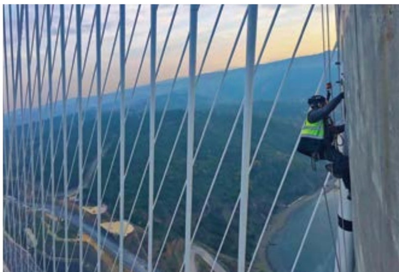
Fig. 4: Inspection and maintenance of the pylons on the Yavuz Sultan Selim Bridge in Istanbul, Turkey by an IRATA-certified rope access technician. Photo courtesy of Yusek Isler.
