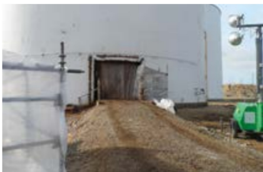
Fig. 4: A garage-door-sized opening was cut into side of the Behemoth to provide interior access for vehicles, including scissor lifts, for the interior tank lining, inspection and associated work.
