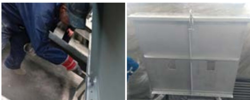
Fig. 13: Stripe-coat application of novel IMM 1 on process vessel wall (left) and finished vessel wall (right).
