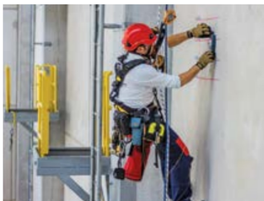
Fig. 5: Non-destructive testing conducted by an IRATA-certified rope access technician in Izmir, Turkey. Photo courtesy of MIRA Rope Access.
