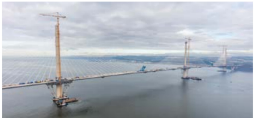
The three-towered cable-stayed bridge spans 1.7 miles, making it the longest of its type in the world.
