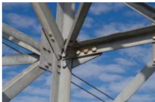
Fig. 3: Galvanized steel has a finite life and in severe environments, rapid depletion of the zinc layers can occur. Methods to increase the film build of the initial HDG can have substantial rewards, especially if augmented with soundly engineered organic coatings.
