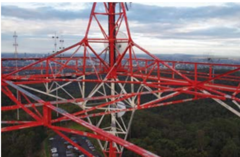
Fig. 2: The structural complexity of an erected lattice mast makes through-life recoating or maintenance very difficult and expensive. It is preferred to engineer in the desired durability by the use of sound galvanizing and compatible high-performance coatings applied prior to assembly and erection.
