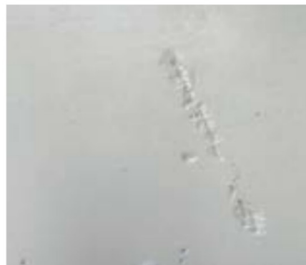
Fig. 5: Thin-film concrete coating in the field, Spalls are coated but pinholes remain.
