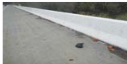
Fig. 11: The 2016 condition of thin-film (two-coat epoxy primer) concrete coating applied in 2004.
