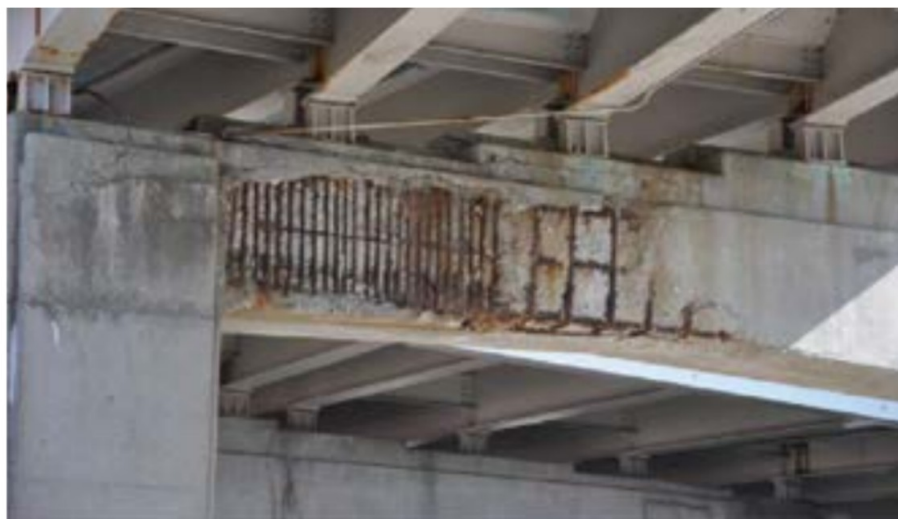
Fig. 1: Deteriorated pier cap under a leaking expansion joint. Figures courtesy of the authors.
