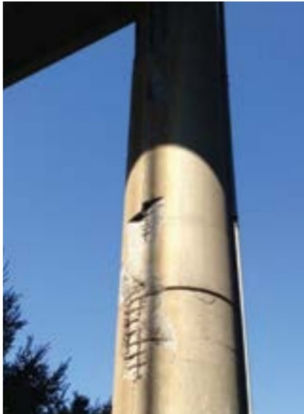
Fig. 2: Deteriorated pier column under a leaking expansion joint.
