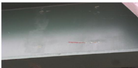
Fig. 4 (Top): This figure shows a shipping and erection defect. Fig. 5 (Bottom): This gouge goes down to substrate and must be repaired to ensure that the coating has the longevity it was designed for.
