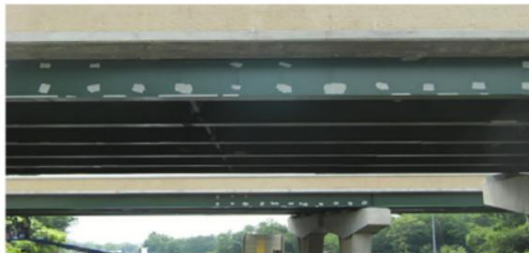
Fig. 6: Applying an additional coat of finish may be necessary to give these fascia defects a uniform appearance after erection is complete.
