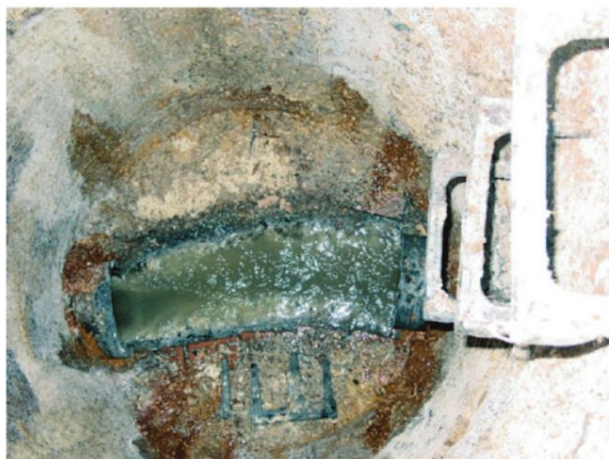
Fig. 4: Manhole structures tend to deteriorate over time due to exposure to a variety of corrosive materials.
