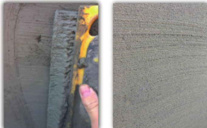
Fig. 3: Spraying and hand-troweling a stand-alone calcium aluminate mortar has proven to be a sufficient long-term repair for manholes not subjected to significant corrosive attacks.
