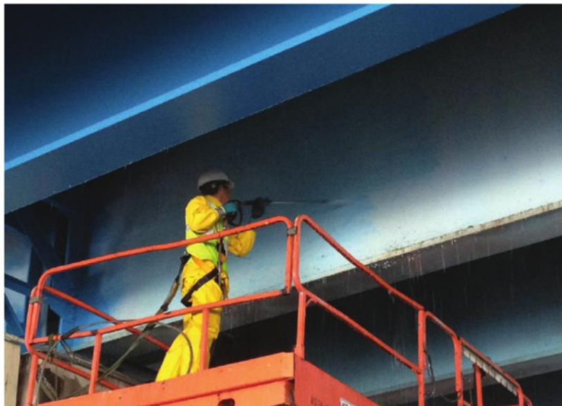
Fig. 2: Low Pressure Water Cleaning (LPWC) being done on a Florida Department of Transportation project to meet SSPC-SP WJ-4/NACE WJ-4, "Light Cleaning."
