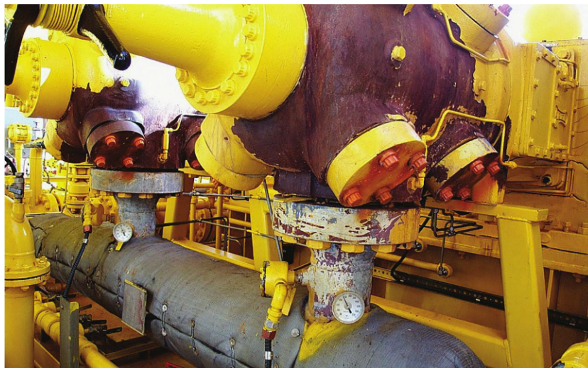
Large areas of the recently applied three-coat maintenance paint failed down to the substrate, exposing bare steel.
