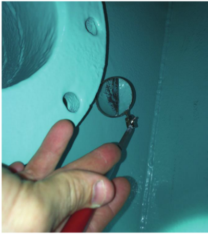
Fig. 3: It was determined primarily through visual inspection that the coating was overall properly installed and free of holidays. This photo shows an improperly applied 100-percent-solids epoxy system that required touch-up.
