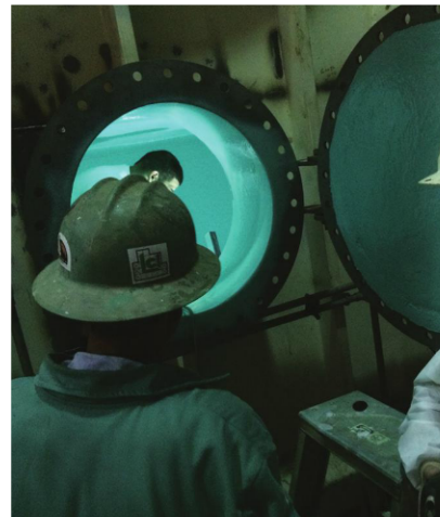
Fig. 4: This is a 24-inch manway leading to sound, hard and well-preserved coating. Roughly 4 inches above the tank floor, the coating began to feel soft.
