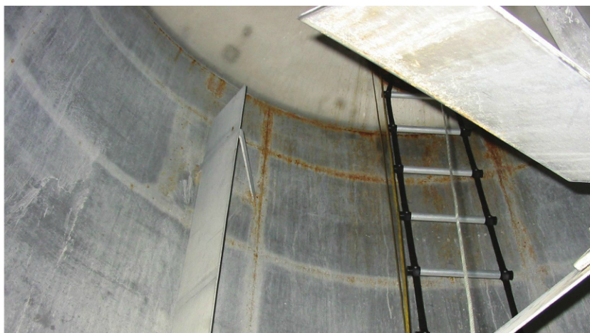
Fig. 2: A view looking up from a 24-inch manhole in a similar tank, exhibiting side baffles and a center mixer. The coating on the side baffle near the top of the tank had softened and showed signs of wear.
