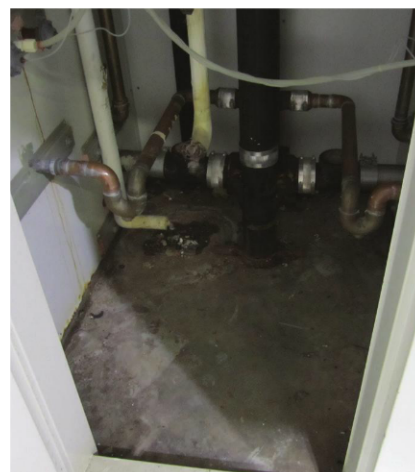
Fig. 2: It is imperative to locate the source of even small leaks as they can often lead to significant moisture issues within a coating system.
