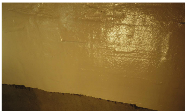
Fig. 4: Although acceptable testing conditions could not be met prior to coating a new concrete wet well, an inspection two-and-a-half years later revealed no moisture-related failures.
