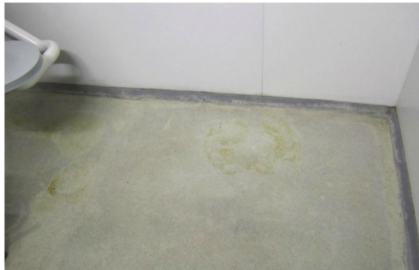
Fig. 4: This photo shows evidence of standing water which has stained the cell floor. Cracks in the coping around the base of the walls allow the water to enter.
