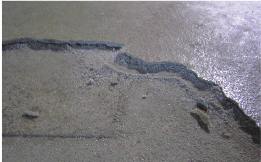
Fig. 3: The failure mechanism also suggests areas without a durable substrate.
