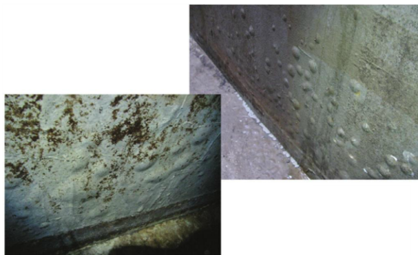
Fig. 3: Within about one year after coating, widespread liquid-filled blisters appeared in the wall of a new concrete pipe gallery that had reported acceptable MVER test values.
