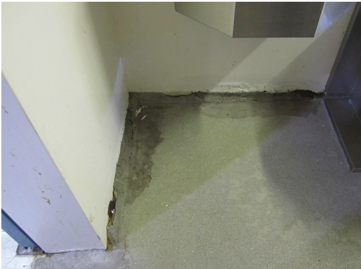
Fig. 1: This photo demonstrates that not only are there cracks and delamination present, but it provides clear evidence of water intrusion. The visible rust stains are only found when ferrous metals begin to corrode. All figures courtesy of the author.
