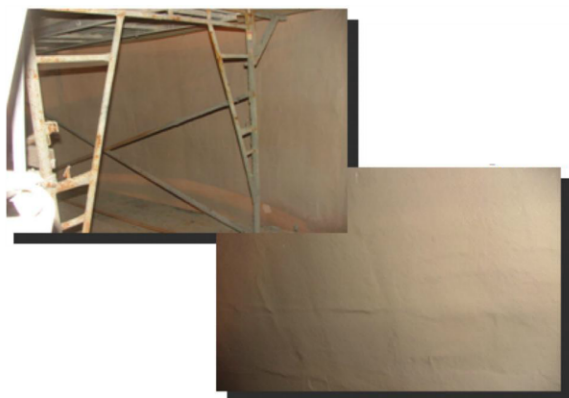
Fig. 2: An inspection of a below-grade channel two years after coating showed no blisters or other moisture-related deficiencies. Lining application of the epoxy glaze coat is shown on the left and the lining after completion on the right.
