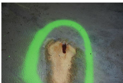
Fig. 5 (Top): Liquid oozing from what appeared to be a compromised area along a seam in the floor.
