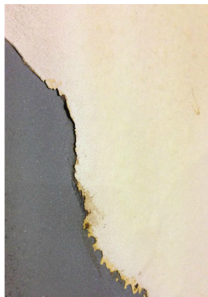
Fig. 11 (Top left): As the coating was peeled back, copious amounts of liquid appeared.
