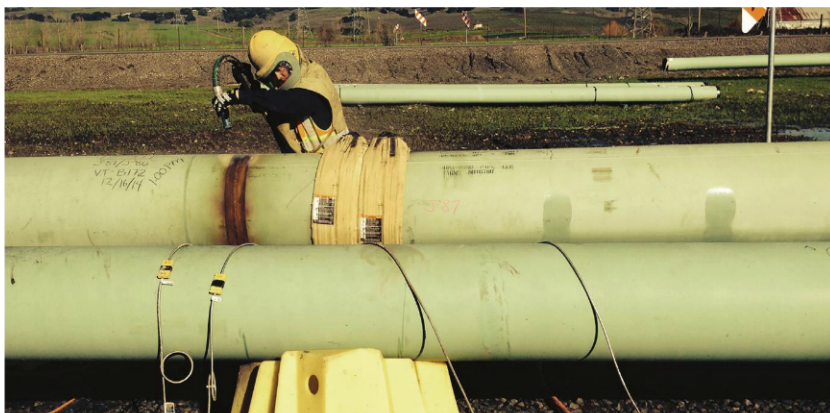
Fig. 5: Abrasive blasting of the heated girth weld. Note that blankets have been moved to avoid damage.
