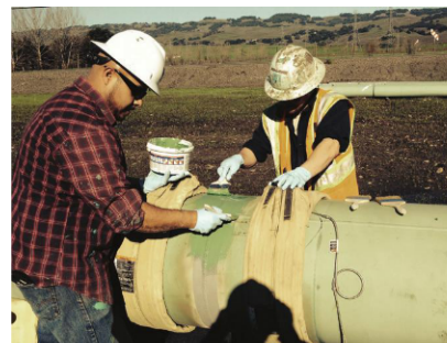
Fig. 6: Heating blankets are reinstalled for coating application and cure.
