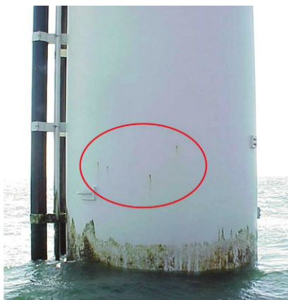
Fig. 2: At the Horns Rev 1 (HR1) facility, pin-point corrosion is noted on TPs painted with the lean two-coat epoxy system. Photo courtesy of FORCE Technology.
