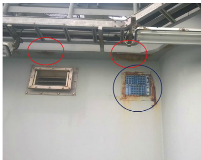
Fig. 7: This image shows an offshore transformer station. Two typical faults in the surface treatment process that initiate corrosion attacks are noted. The red circles show the lack of rounding of edges (chamfering) on part of the steel bar. The blue circle shows a poorly mounted and painted light accessory after installation of the station. The intact ventilation duct on the left side of the photo has been mounted correctly during the manufacture of the station. Photo courtesy of Dong Energy.
