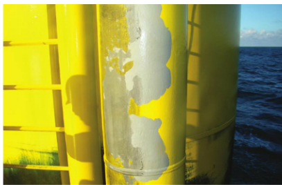
Fig. 8: The flaking of the topcoat and the penultimate intermediate coat on this boat landing was caused by aluminum dust originating from an adjacent thermal spray application during construction and from exceeding recoating intervals. Photo courtesy of FORCE Technology.
