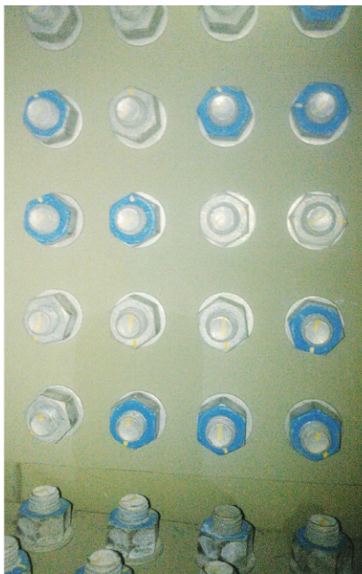
Fig. 1: The two bottom rows of bolts show damage to the galvanizing caused by tightening with too large of a socket.
