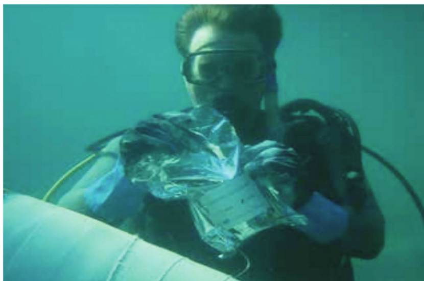
Fig. 4: Underwater application of composites. Note the prepackaged, pre-impregnated resin system.
