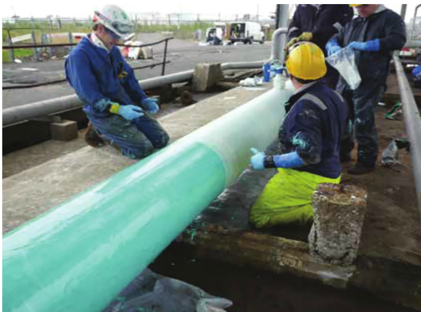
Fig. 2: Installation of a composite coating system.
