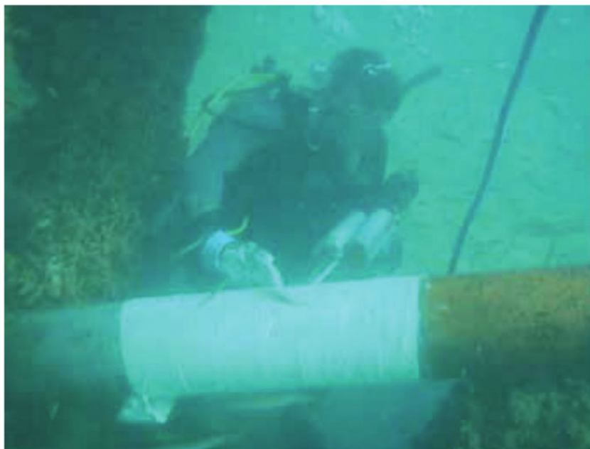
Fig. 5: View of underwater application of composites.
