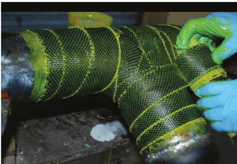
Fig. 3: View of the application of an epoxy/carbon fiber system repair of a T-section.
