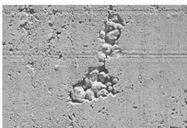
Fig. 1: Performing a concrete condition assessment can expose the presence of bugholes, honeycombs or cracking prior to coating application. Photos courtesy of SSPC.
