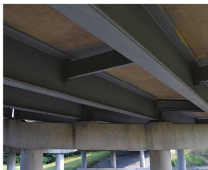
Fig. 3: Bridge rated very good with MCU three-coat systems and concrete deck.
