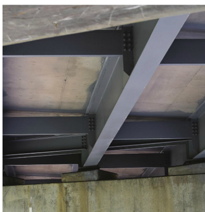
Fig. 4: PAS two-coat coating system with a concrete deck. This bridge was rated very good.
