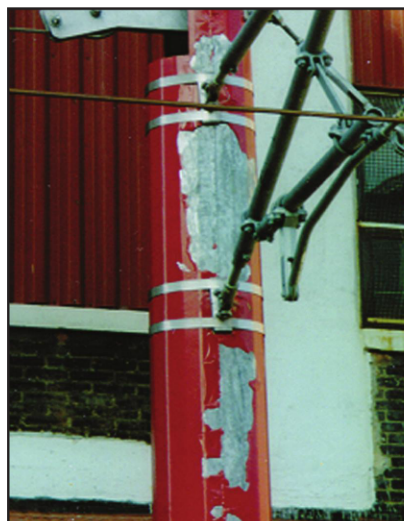
Fig. 4: Galvanized pole with peeling paint.
