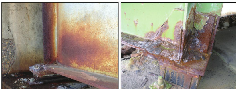
Fig. 3: Sample photos from the MNDOT "Steel Bridge Coating Condition Assessment Photographic Field Guide," developed to assist with performing coating condition assessments.
