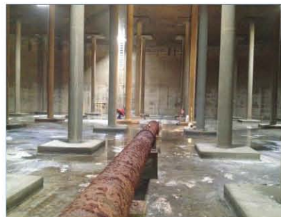
Fig. 5: Accelerated corrosion of the ductile iron pipe surfaces prior to contract. Note stainless steel anchor bolts on pipe support (right). Photos courtesy of Carl Bowers, Amos and Associates.
