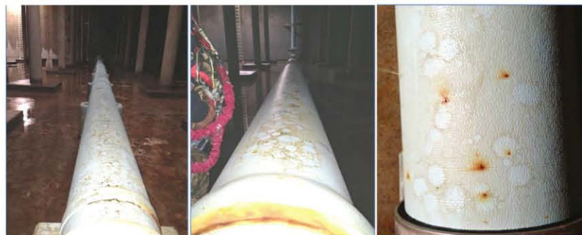
Fig. 6: Existing DI pipe (left) and new pipe at the one-year inspection (center and right). Photos courtesy of Carl Bowers, Amos and Associates.
