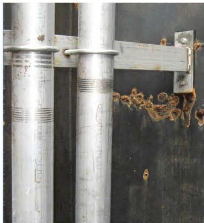
Fig. 4: Bare stainless steel piping and support brackets bolted to coated carbon-steel tank wall. Photo courtesy of the authors.
