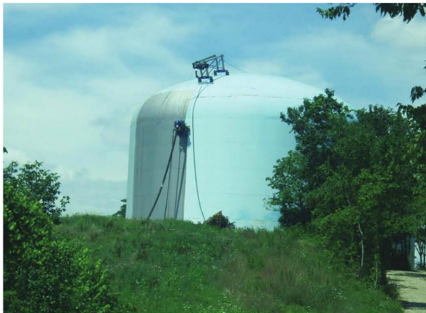
Robotic blasting equipment preparing exterior surfaces for coating. Photo courtesy of Tank Industry Consultants.
