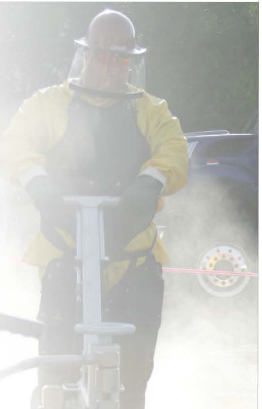
Fig. 1: Semi-automated "mower" style waterjet cleaning and prepping horizontal surfaces. Photos courtesy of WJTA-IMCA.
