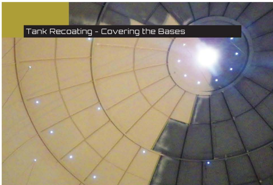
View of interior roof and support system with rigging couplings in place. Photo courtesy of Tank Industry Consultants.
