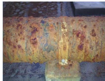
Fig. 5: Accelerated corrosion of the ductile iron pipe surfaces prior to contract. Note stainless steel anchor bolts on pipe support (right). Photos courtesy of Carl Bowers, Amos and Associates.
