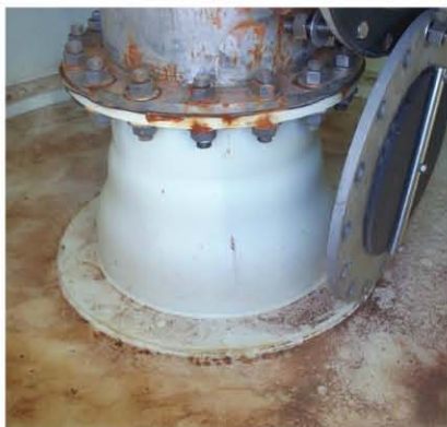
Fig. 3: Stainless steel mixing system bolted to the carbon-steel inlet/outlet piping. Photo courtesy of Andrew Kirby, PE.
