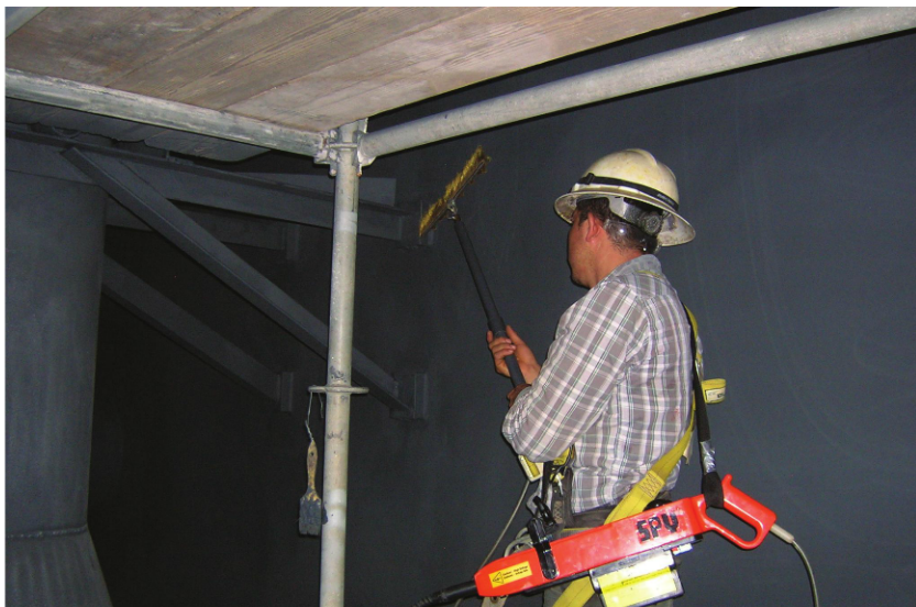
The Tank 2003 side shell and floor were 100-percent high-voltage holiday detector-tested after application and curing of the second coat of vinyl ester lining.
