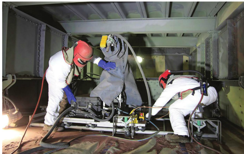
Workers slide the robot into position for the next blast. Photo: Roads and Maritime Services (RMS)
