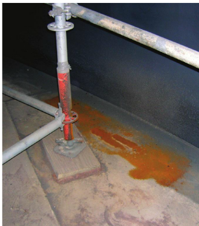
Because of effective dehumidification, small amounts of rain leakage on the blasted tank floor did not "turn" adjacent areas of white metal blast. The small rusted areas were reblasted.
