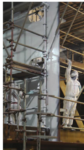
Third and final system coat being applied.
