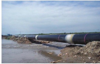
The fiberglass-plastic-protected field joints.
