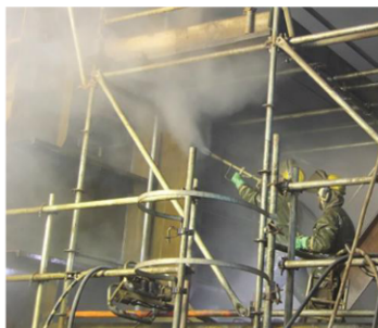
Second system coat being applied (top left), electrically operated UHP waterjetting machines working at 40,000 psi (top right) and worker waterjet cleaning to SSPC-SP WJ-2/ NACE WJ-2 standard (above).
