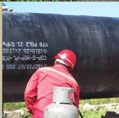
Applying the resin to the fiberglass wrap (right) and the finished field joint to be protected (above).
