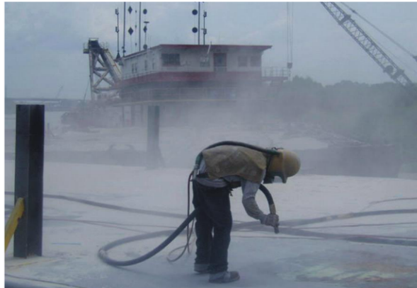
During the blasting of surfaces, high humidity can cause flash rusting to occur before prime coats are applied.
