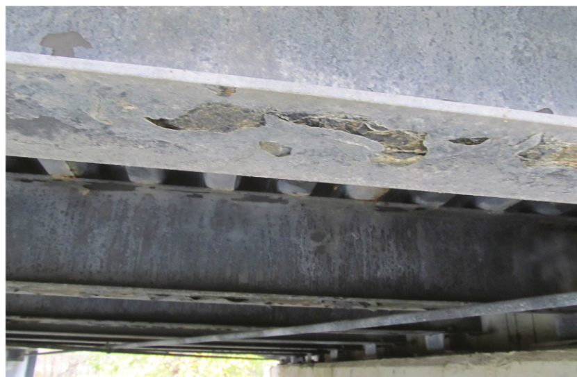
Fig. 2: The galvanized zinc layer was cohesively delaminating along many stringer and floor beam flanges. Delamination typically occurred in areas where surfaces had heavy white corrosion deposits.
