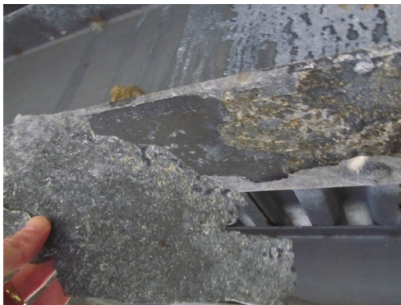
Fig. 3: Large pieces of delaminating zinc could be removed from members with a thin layer of galvanizing remaining on the steel.
