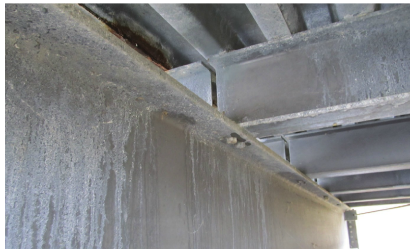
Fig. 1: Galvanized members display white zinc corrosion product on surfaces. Other areas are a uniform dark gray color that is characteristic of galvanizing on reactive steel. All figures courtesy of KTA-Tator, Inc.
