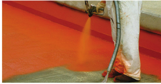
Fig. 2: Spray application of bridge deck membrane.
