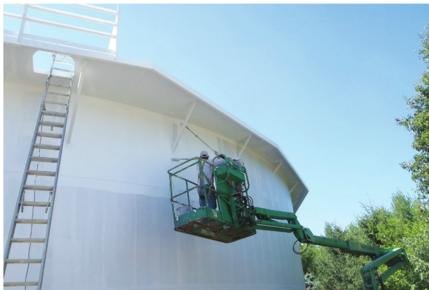
Coating the tank exterior.
