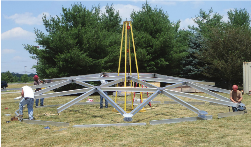
(Above and below right) Assembling the new geodesic aluminum tank roof.
