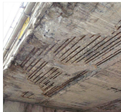
Fig. 1: Concrete bridge deck corrosion.
