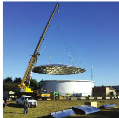
Positioning the new roof over the tank.
