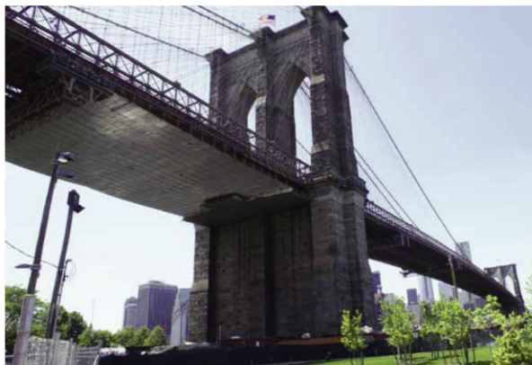
Dealing with traffic, existing lead coatings and coordination with outside agencies were some of the challenges in painting the 132-year-old Brooklyn Bridge. Photos courtesy of New York City DOT.
