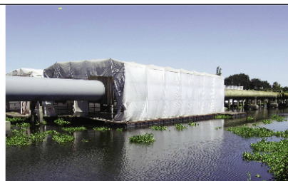
Floating containment structures were utilized to capture existing lead-based coatings while recoating above-ground, over-water portions of the Mokelumne Aqueducts. Photos courtesy of Mark Lewis, East Bay Municipal Utility District.
