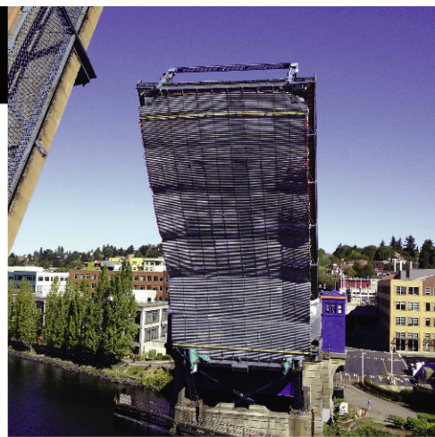
Contractors painting the Fremont Bridge had to clear the bridge to allow it to open for marine traffic nearly three dozen times per day. Photos courtesy of Seattle DOT.
