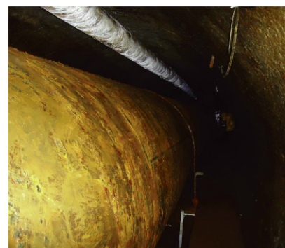
Contractors faced several challenges cleaning and recoating a 1,750-foot-long penstock located 80 feet underground at the Mamquam Generating Station. Photos courtesy of Certified Coating Specialists Inc.
