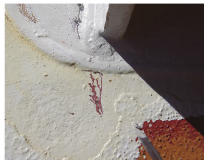
Figs. 5 and 6: The replacement valve has been diligently painted (top), but with what proved to be an alkyd enamel. This column base was one of many coated with multiple layers of polyurethane, but all without the Part B added (bottom).
