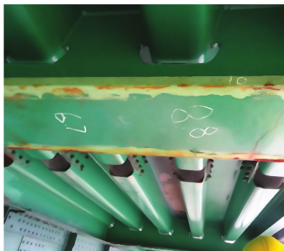
Fig. 2: Edge coating should include a stripe coat, even for spot repairs.
