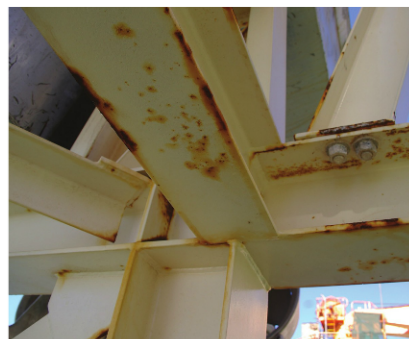
Fig. 2: An onshore-coated steel fabrication now fitted to an FPSO that was inadequately coated for offshore service. The DFT measured around 3.5 mils (90 microns). Predictably, little resistance to marine exposure was provided.
