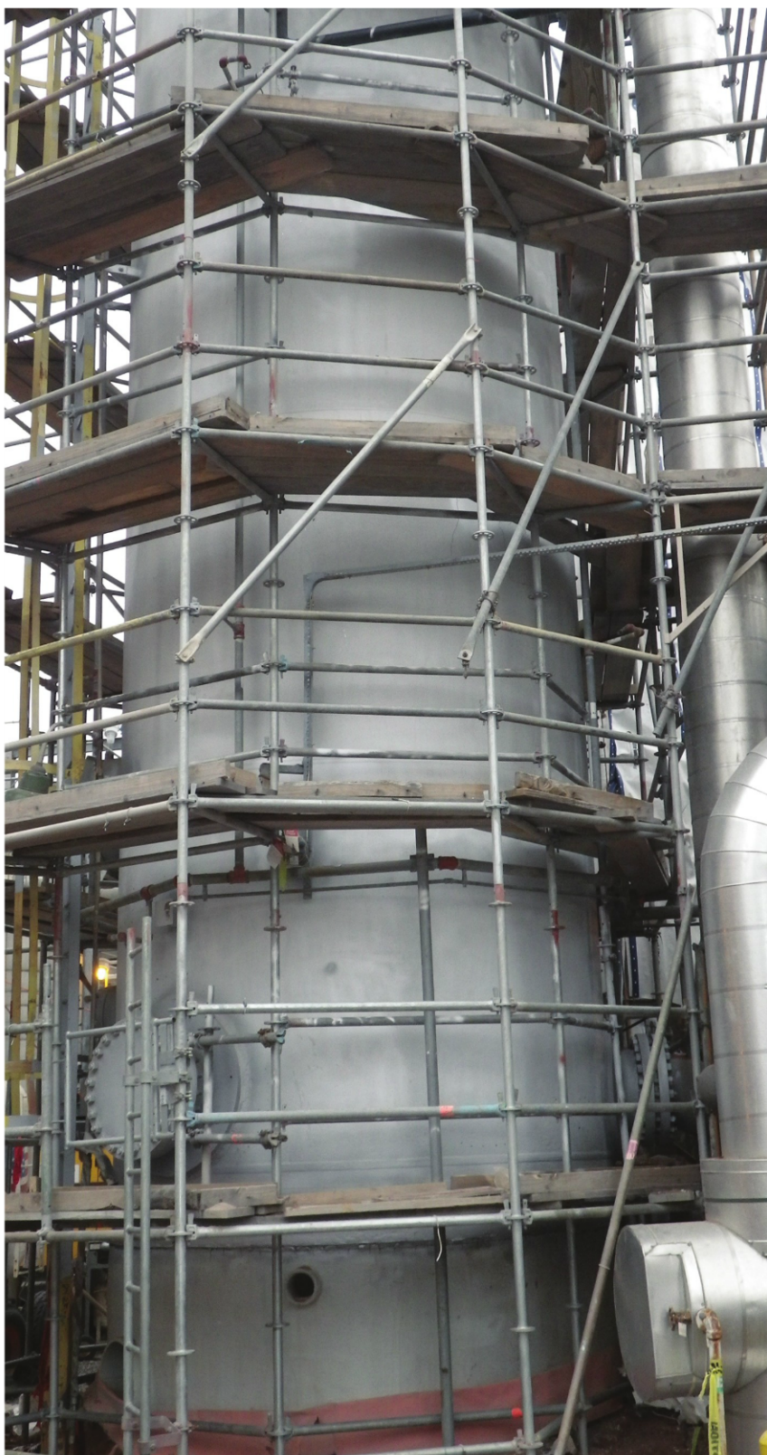
Fig. 1: Multi-story process vessels provide large relatively flat areas for arc-sprayed thermal spray aluminum. The high cost of lost production on such vessels offsets the higher application cost of thermal spray because of the shorter return-to-service time.
