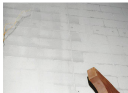
Fig. 3: Pattern of moisture on the interior of the block walls.
