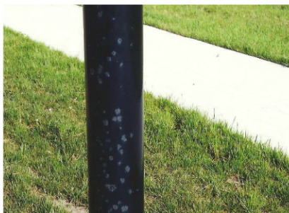
Fig. 5: Paint failure near the base of a light pole. The failure was essentially confined to only one side of the pole, from ground level to about 7 feet.
