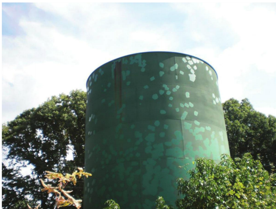
The aesthetics of a field touch-up can be compromised when the touch-up paint does not closely match the color of the weathered original coating. Courtesy of KTA-Tator, Inc.
