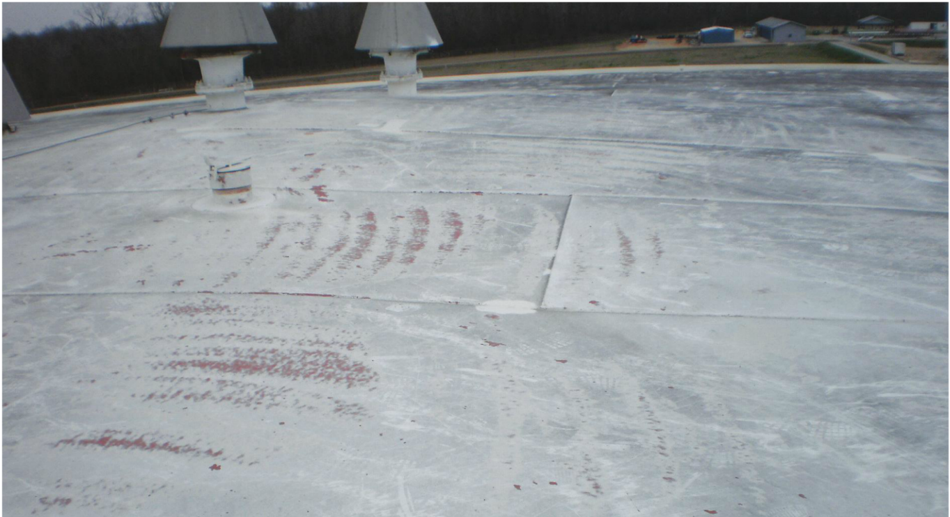
Severe chalking and erosion of an epoxy coating caused by degradation of the resin in ultraviolet light. The degradation resulted in both aesthetic and performance problems. Courtesy of KTA-Tator, Inc.
