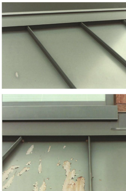
Fig. 1 (top): Panels adjacent to brick, showing no failure. Fig. 2 (bottom): Panels adjacent to a window a few feet away from the panels shown in Figure 1. Note the extensive paint failure.
