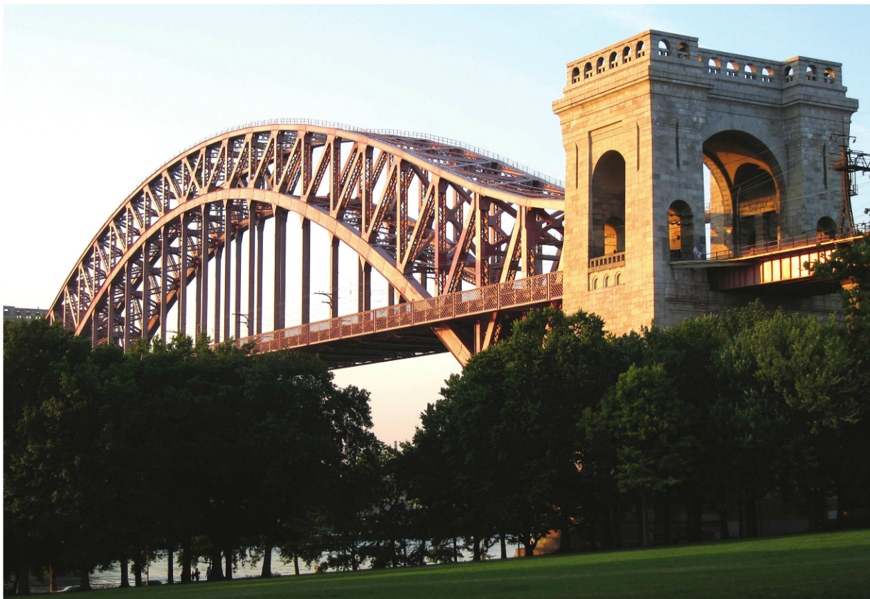
The red topcoat on the Hell Gate Bridge experienced severe fading as result of insufficient clear coat application.
