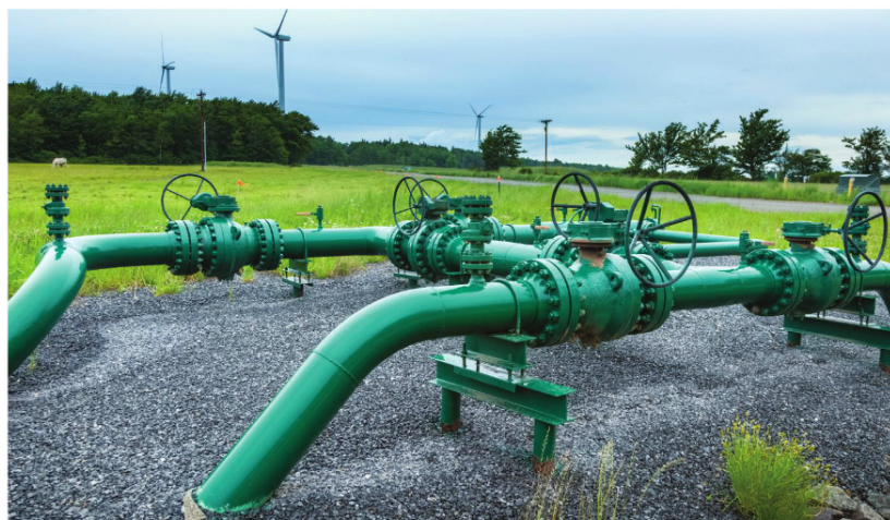
Fig. 3: Air to soil transition on a pipeline run. © iStockphoto.com/drnadig
