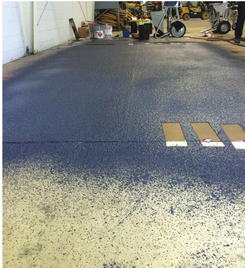
Fig. 3: An epoxy non-skid deck coating successfully applied with a two-ball piston pump. Photo courtesy of C.H. Reed.
